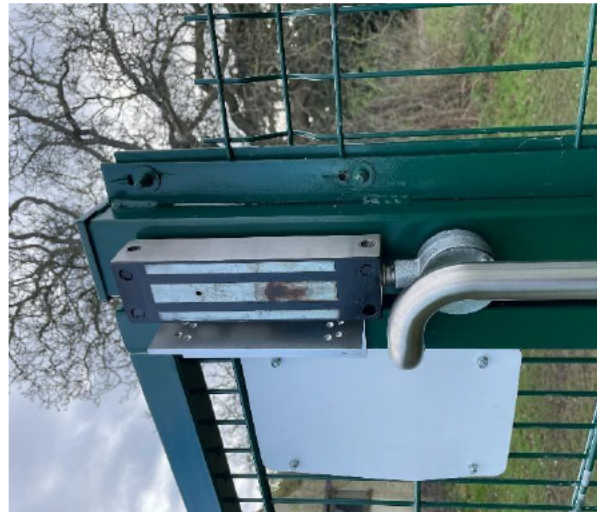
Magnetic access control lock stolen from gate 09/12/2021 to prevent automatic locking during normal school use.
