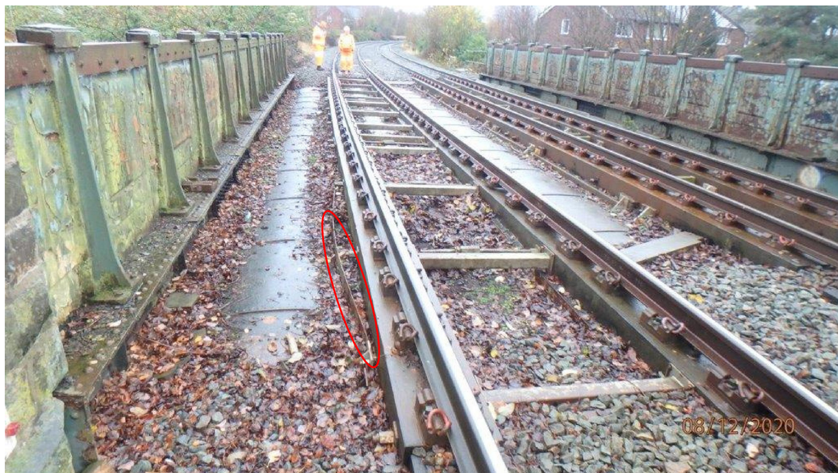
Figure 20: The leading section of the down line on bridge 3 observed during a structure examination in December 2020 showing the bowed steel strip and the location of the missing cleat (courtesy of Network Rail with RAIB annotations).
