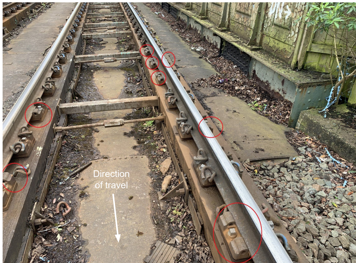
Figure 26: The LBS as observed during a bridge examination report in April 2024 showing the missing rail clips at the north end of the down line (courtesy of Network Rail with RAIB annotations).
