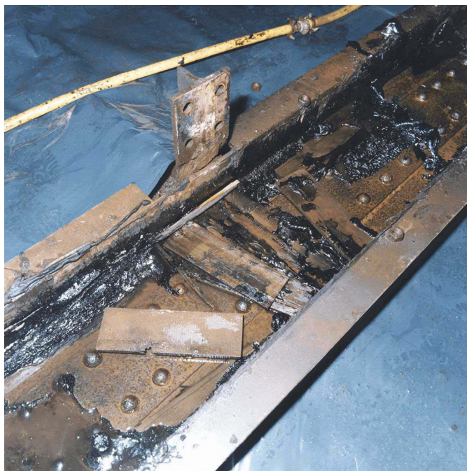
Figure 36: Failed 1997 LBS installation at Althorpe (from business process document NR/SP/TRK/9003 courtesy of Network Rail).
