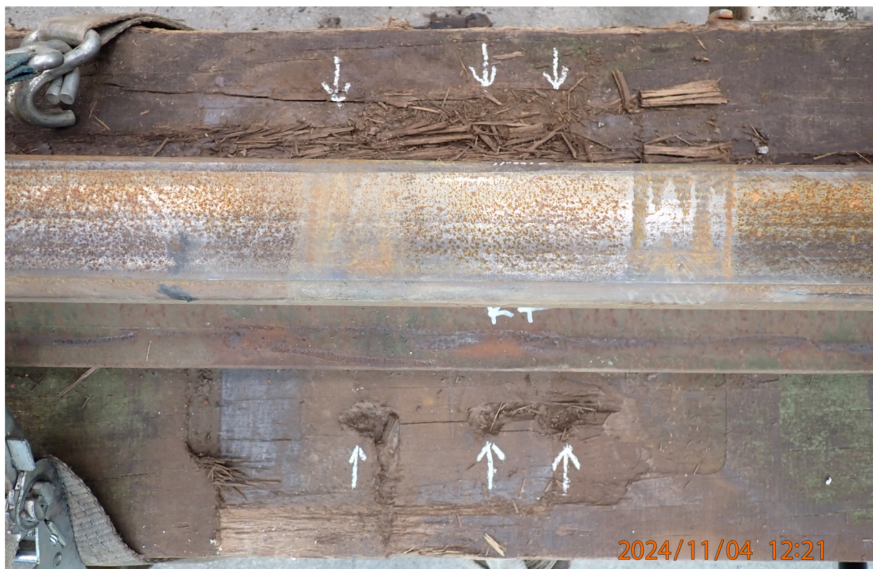
Figure 13: The R7 baseplate position showing evidence of previous screw holes.
