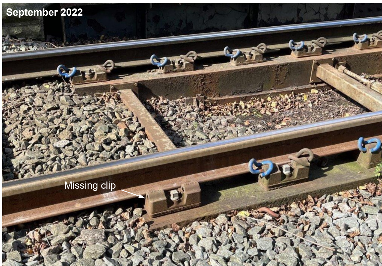
Figure 23: The presence of additional clips on the baseplates and missing clips from the baseplate at position R1 observed during a structure examination report in September 2022 (courtesy of Network Rail with RAIB annotations).
