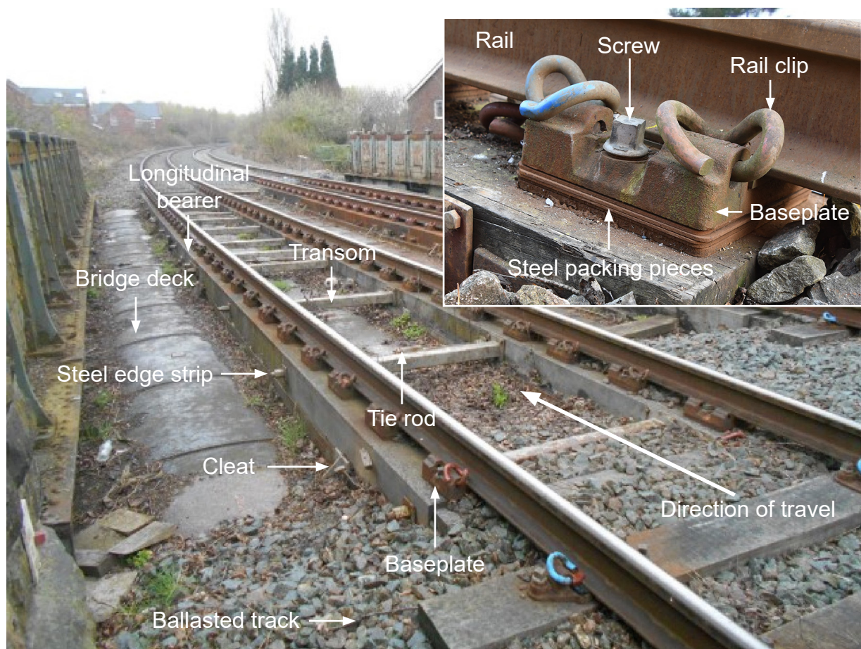
Figure 6: The main components of the LBS of the Down Crowthorne line on bridge 3 (courtesy of Network Rail with RAIB annotations).
