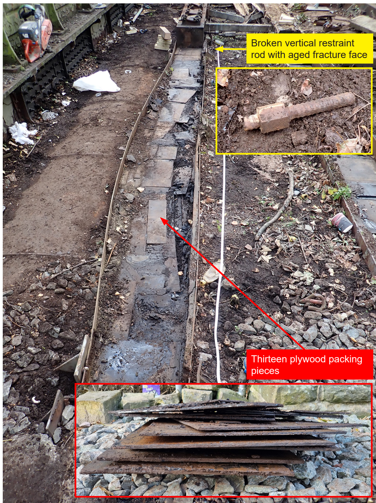
Figure 21: The leading section of the down line cess-side bearer on bridge 3 following removal of the bearer and rail.
