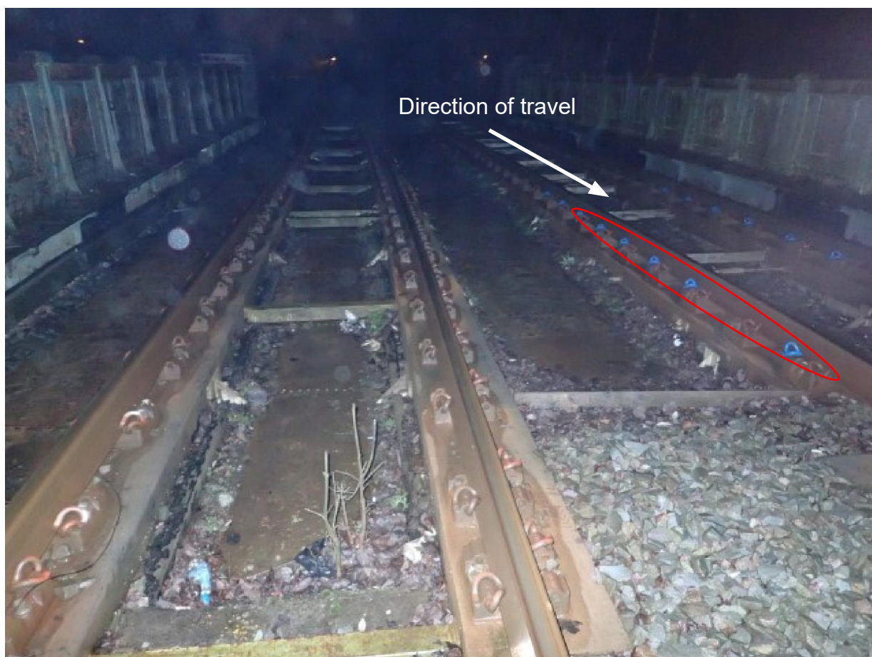
Figure 18: The LBS on bridge 3 during a structure examination in January 2018 showing additional rail clips on baseplates at the north end of the down line (courtesy of Network Rail with RAIB annotations).
