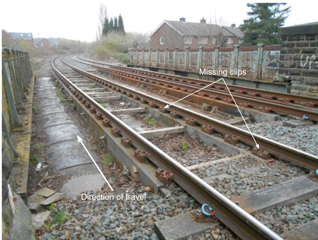
Figure 17: The LBS on bridge 3 during a structure examination in April 2016 (courtesy of Network Rail with RAIB annotations).
