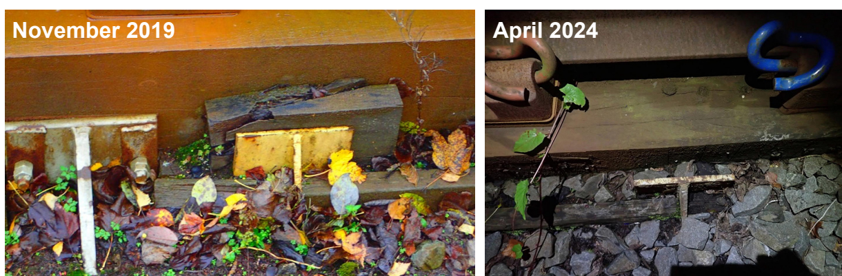
Figure 22: Photographs from structure examination reports on two dates showing the typical states of the wooden wedges between the cleats and the bearer sides (courtesy of Network Rail with RAIB annotations).
