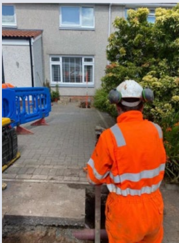
Figure 6: A worker using a mole to unloop a property
