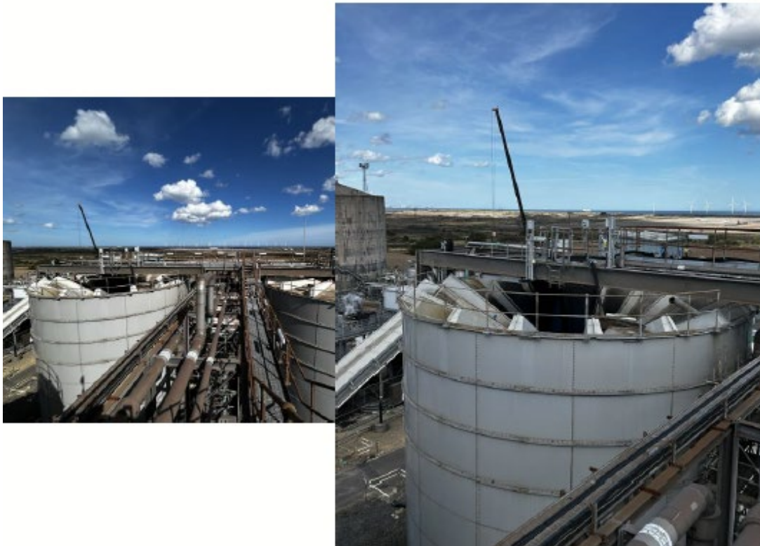
FIGURE 19: COLLAPSE OF GLASS REINFORCED PLASTIC (GRP) STRUCTURE AT BRAN SANDS STW
