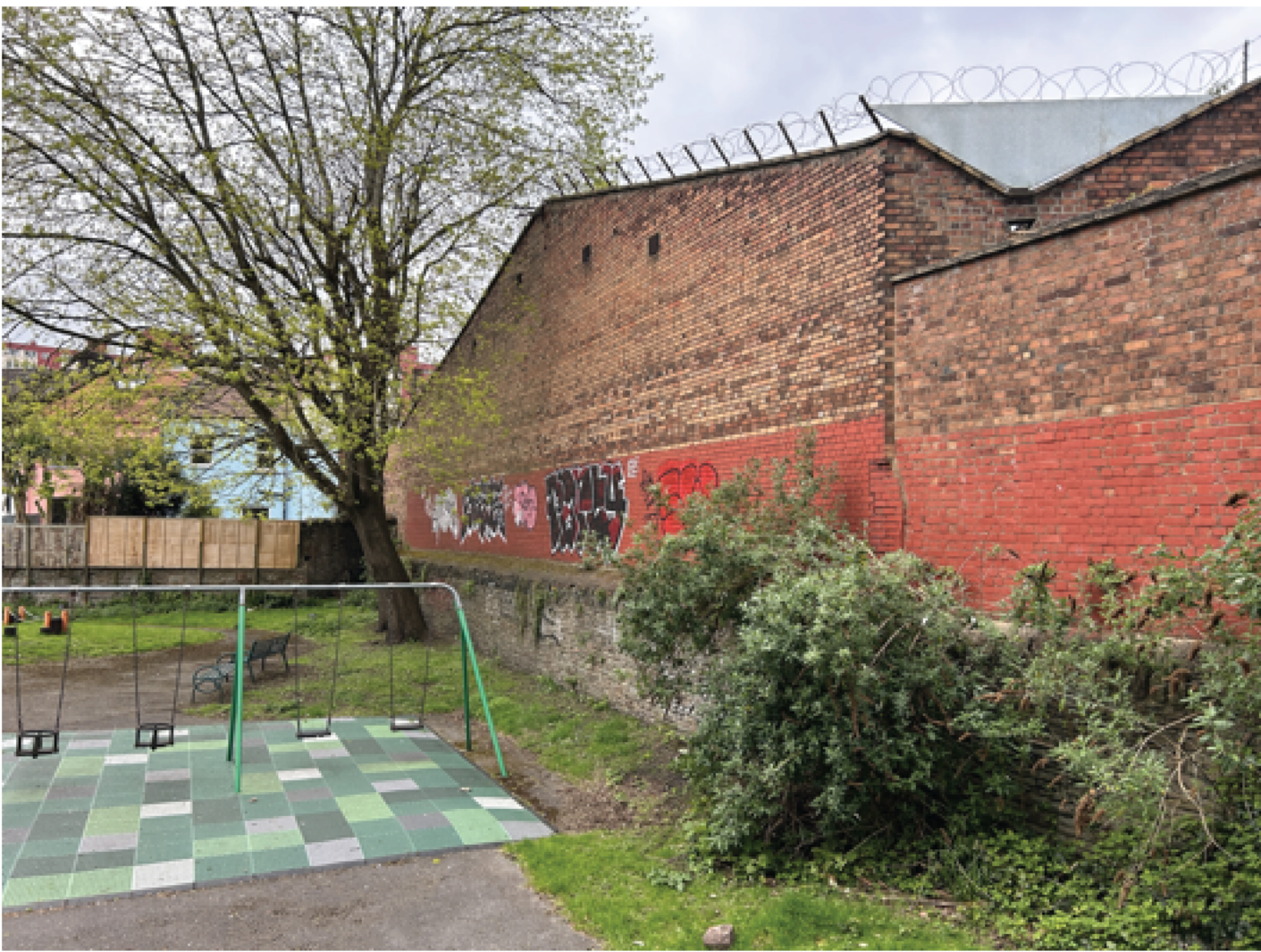
BACK OF EXISTING BUILDING FROM GAUNT'S HAM PARK
