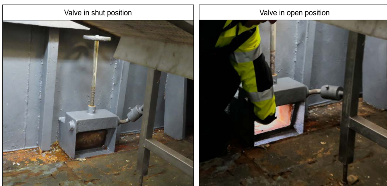
Figure 5: Example tonnage valve
