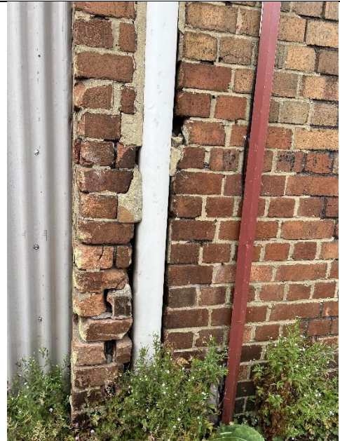
A8 Downpipe to the left of main door had some cracks and crevices
