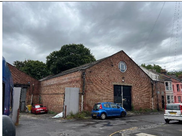
A1 Main elevation. Crevices in brickwork are around the white downpipe seen to the left of the main doors
