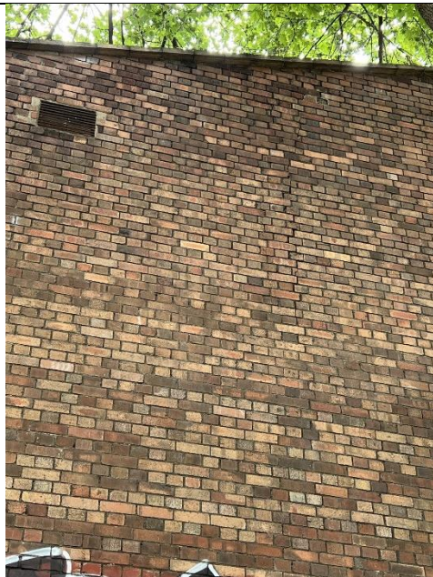
A11 Grill internally covered the air vents to prevent bat access. The crack in the brickwork offers future potential for bats if it enlarges.
