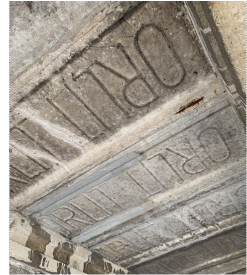
Figure 16: Orlit soffit
