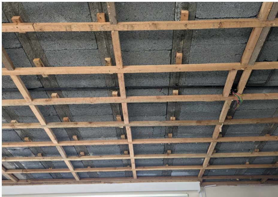
Figure 22: Example of soffit to beam and hollow pot floor
