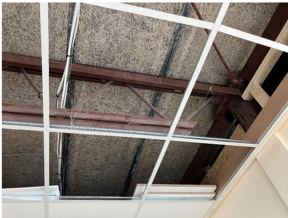
Figure 28 - Woodwool roof slab supported by steel trusses
