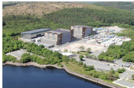
Image above: Trawsfynydd site following reactor height reduction
