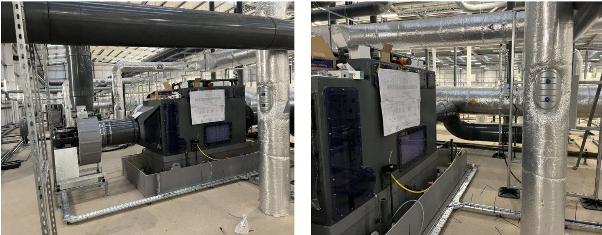
Figure 13: Wet gas scrubber
