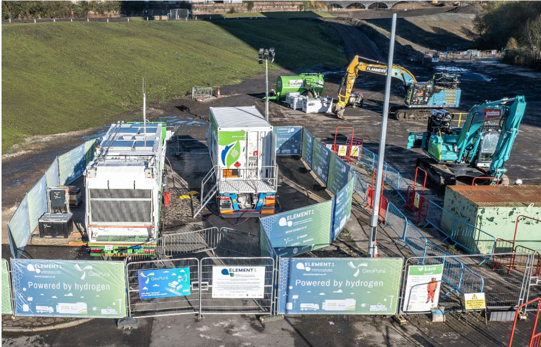
Figure 47 HyTanka® dispensing hydrogen on site in Manchester
