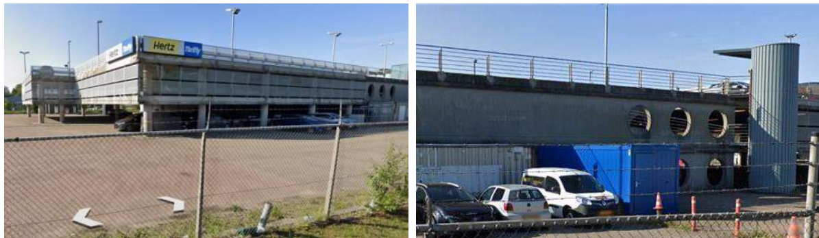
Figure 12. Contemporary images of the elevation of the Schiphol Airport car park taken from Google Streetview
