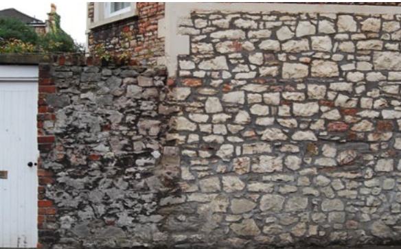
Figure 32: Stone walling materials, Kenilworth Road
