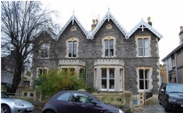
Figure 31: Trelawney Road, Victorian facade with decorative bargeboards
