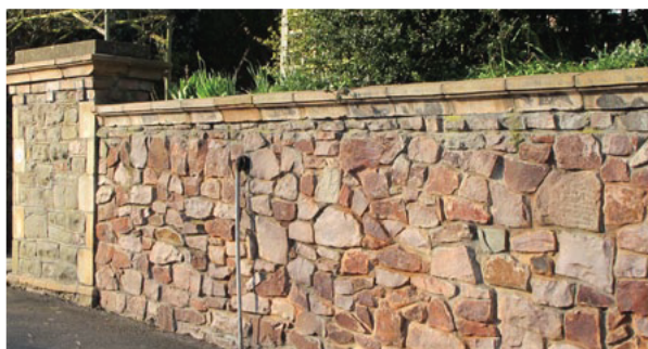
Figure 100: Brandon Hill stone retaining wall, Woodstock Road
