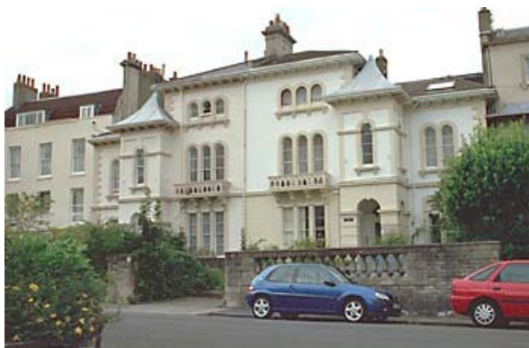
Figure 69: Nos. 71 - 73 Lower Redland Road
