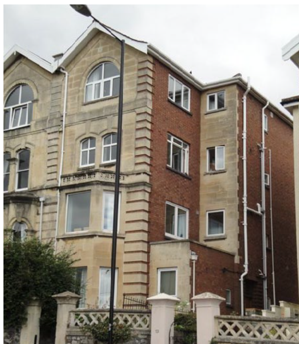
Figure 118: uPVC windows, Redland Road
