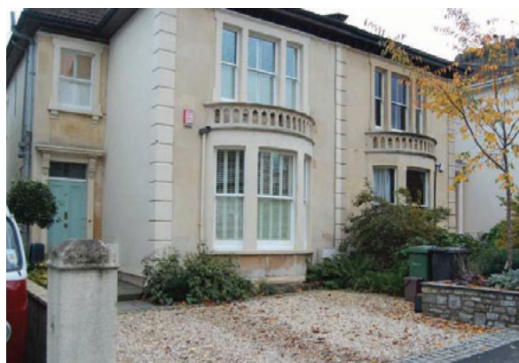
Figure 82: Zetland Road houses
