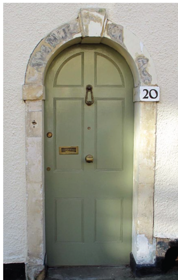
Figure 95: Flush-panel door with limestone surround, Luccombe Hill
