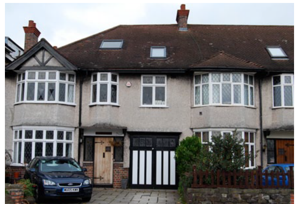
Figure 22: Inter-War houses, nos. 9 - 11 Cotham Lawn Road
