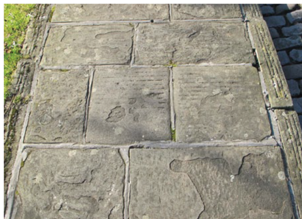
Figure 97: Pennant pavement and kerb, Redland Green
