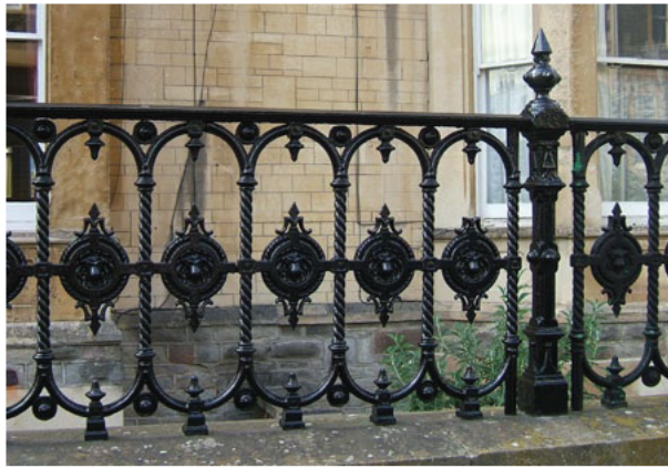
Figure 99: Cast iron railings, Cotham Vale
