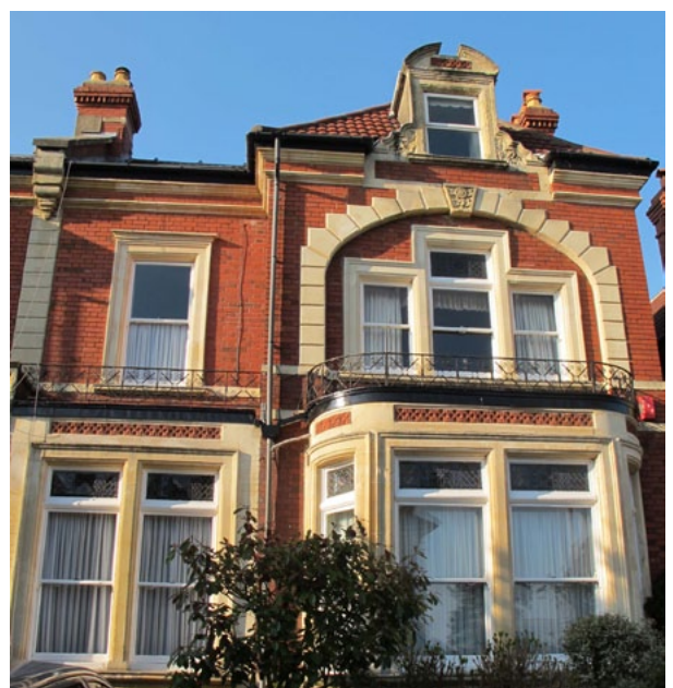
Figure 91: Late Victorian detailing, Woodstock Road
