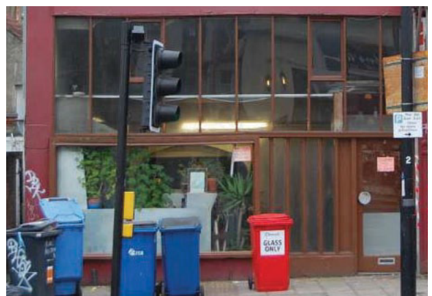
Figure 114: Poor quality shopfront
