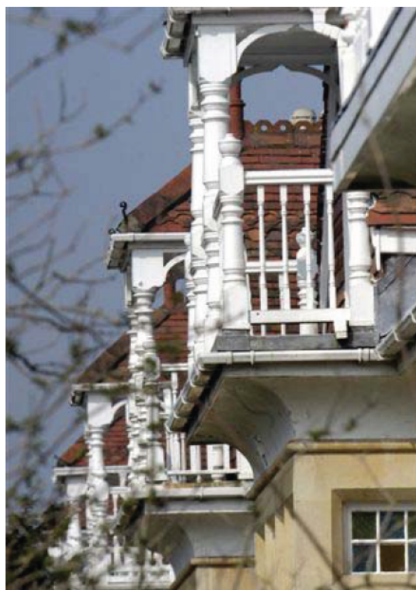
Figure 96: Timber balconies, Cotham Park
