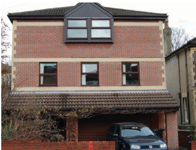
Figure 115: Poorly designed infill
