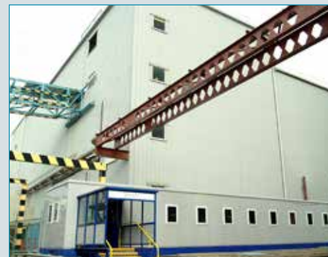
Magnox Reprocessing Plant - Sellafield
