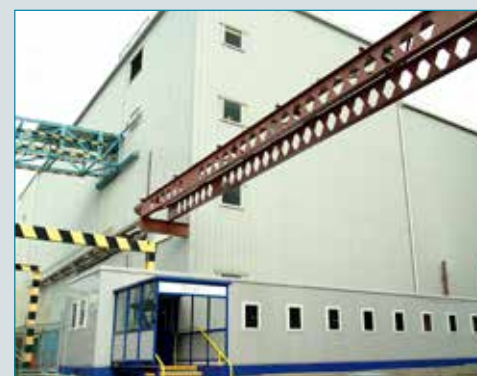
Magnox Reprocessing Plant - Sellafield
