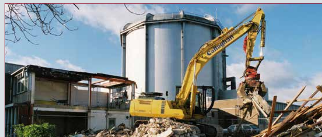
Demolition work at Harwell
