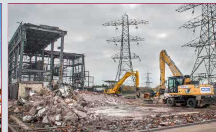
Demolition work at Oldbury
