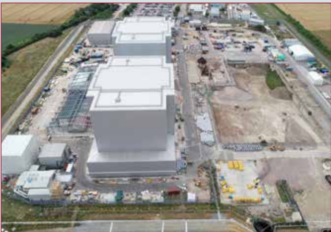
Bradwell in care and maintenance
