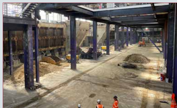
Turbine hall being cleared at Sizewell A
