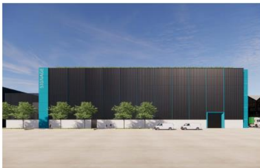
Figure 4 - CD8-001 Soundstage façade facing internal streets, page 57
