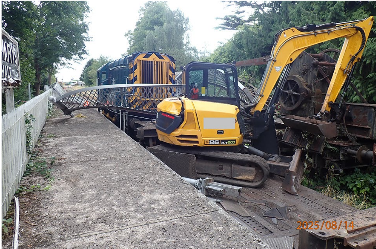
Accident scene looking towards rear of train.
