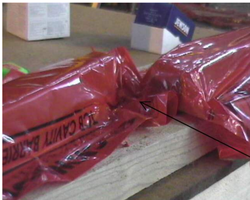
Figure 19 – Discontinuity at the junction between two cavity barriers
