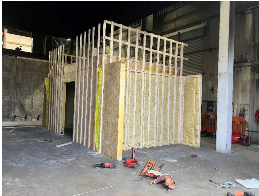
Figure 77 – Timber frame compartment during construction Note that the additional structure above the fire compartment was provided to provide safe access for installers and the BRE team
