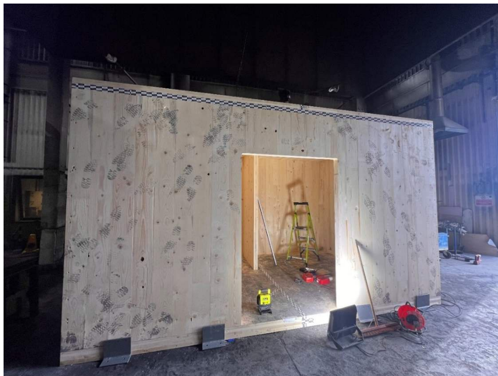
Figure 1 – CLT compartment during construction
