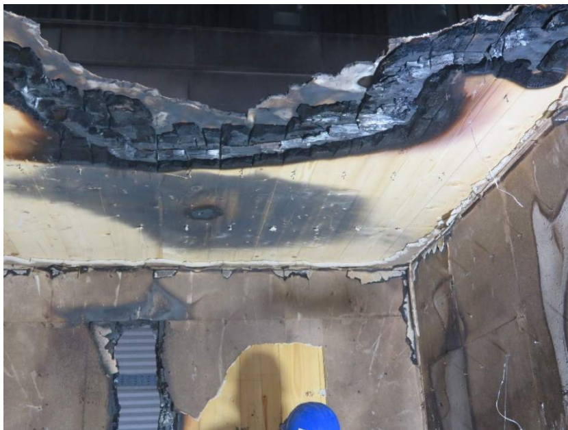
Figure 52 – Consumption of parts of the floors and walls
