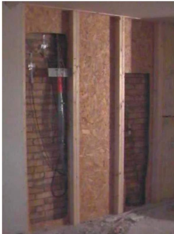
Figure 22 – Internal view of gable end wall with linings removed
