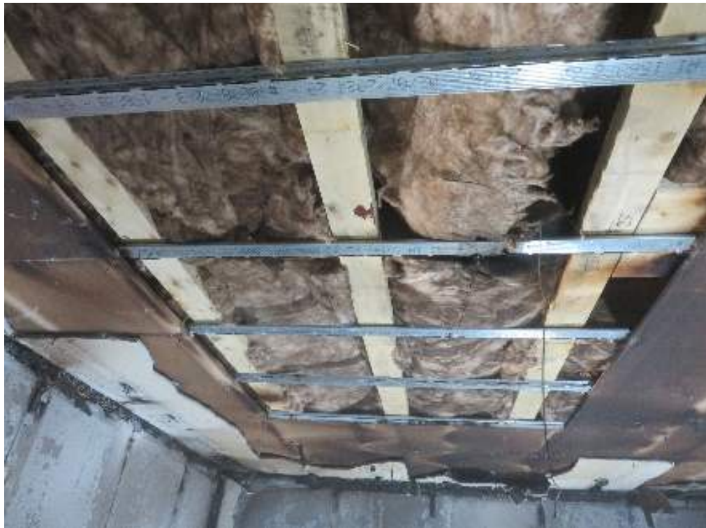
Figure 96 – Engineered Floor Joists following removal of plasterboard linings
