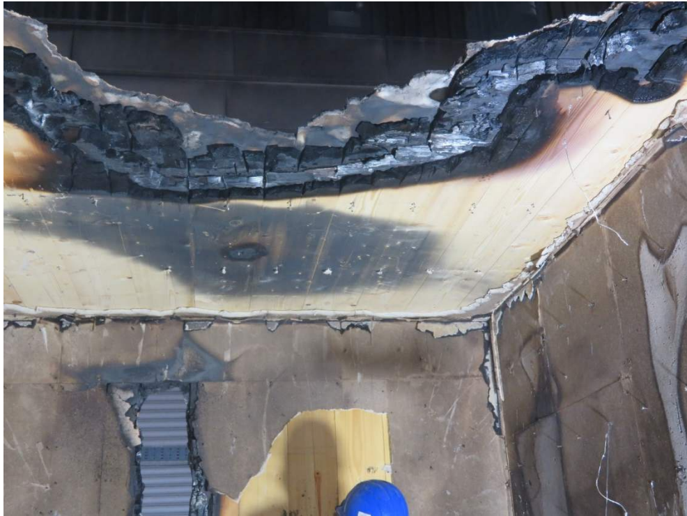
Figure 22 – Charring of CLT roof panel with intact timber beyond the char layer
