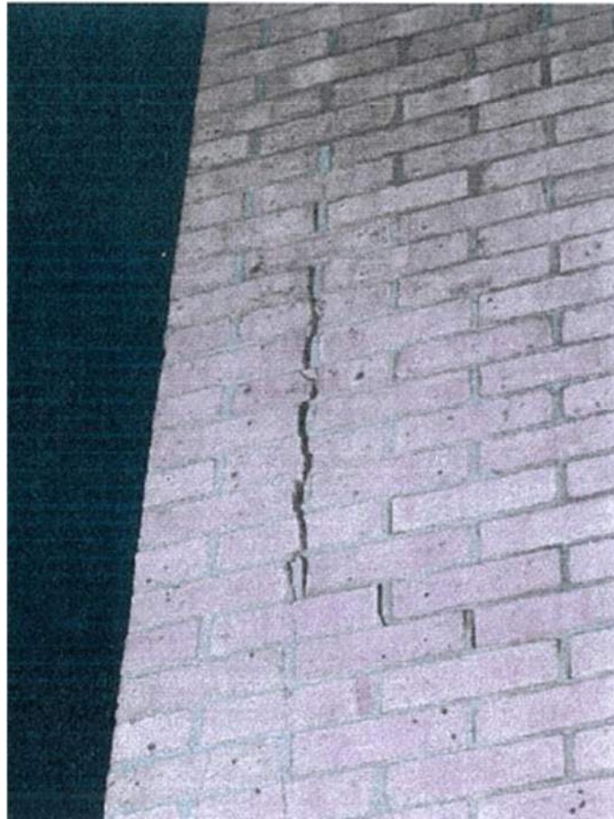
Figure 2 – Cracking in gable end wall at SW corner of the building
