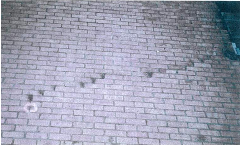
Figure 27 – Cracking in gable wall extending to lower left corner of third floor kitchen window
