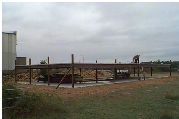
Figure 4 – The open car park configuration used in the tests sponsored by ECSC 14 . This is for the setup in test 1. Note that this appears more like a large car port than a car park.
