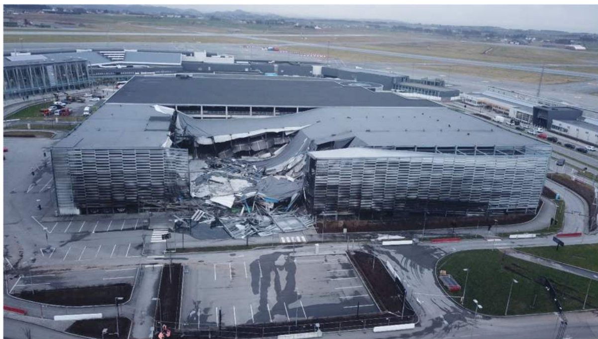
Figure 9 – Aerial photo of the Sola airport car park after the fire, showing the partial collapse 17
