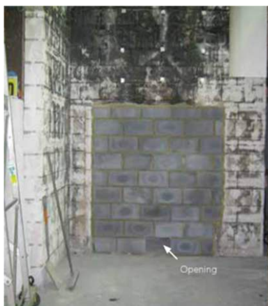
Figure 25 – Cladding wall with hearth bricked in
