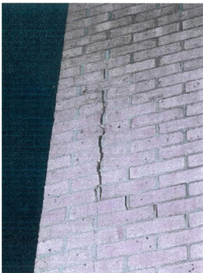
Figure 26 – Cracking in gable end wall at SW corner of the building
