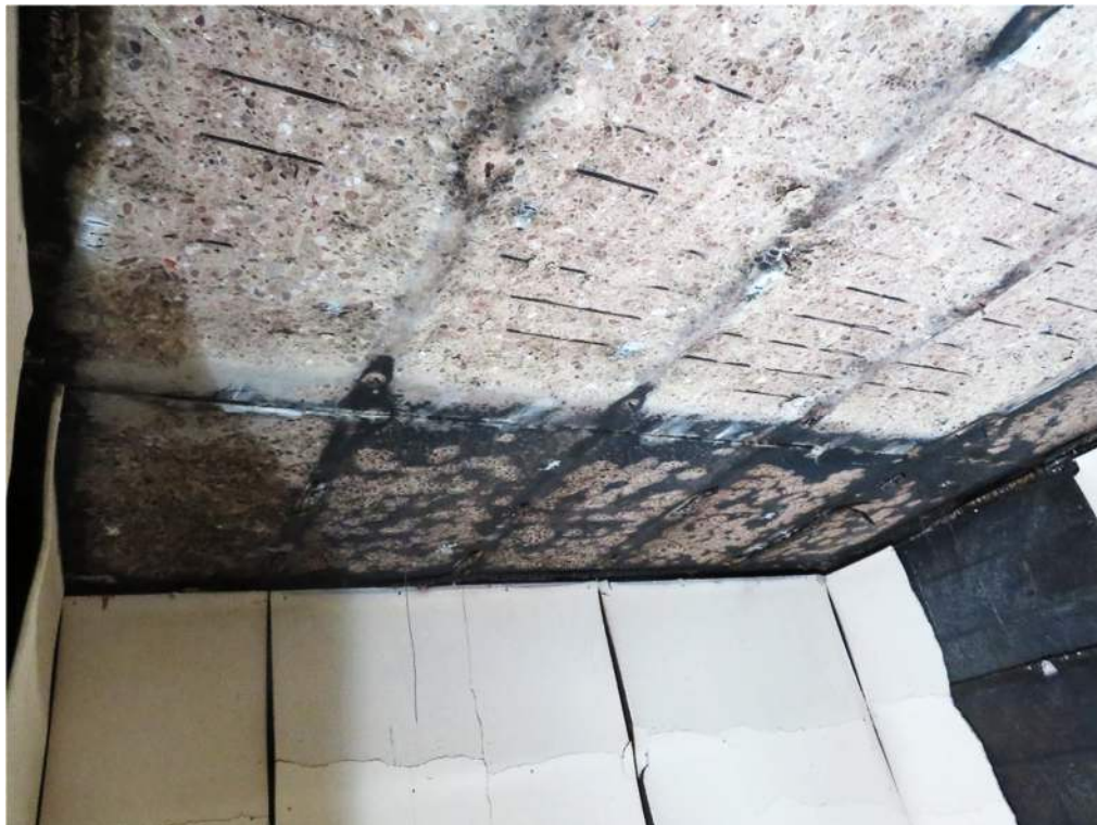
Figure 19 – Post-fire photograph showing extent of spalling to the soffit of the precast floor slabs
