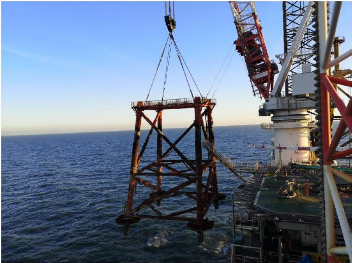
Figure 8.4: Jacket removal
