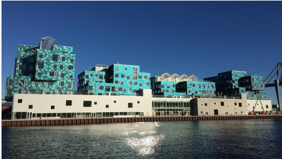
Figure 2. Example of building-integrated photovoltaic panels (BIPV) of the Copenhagen International School
