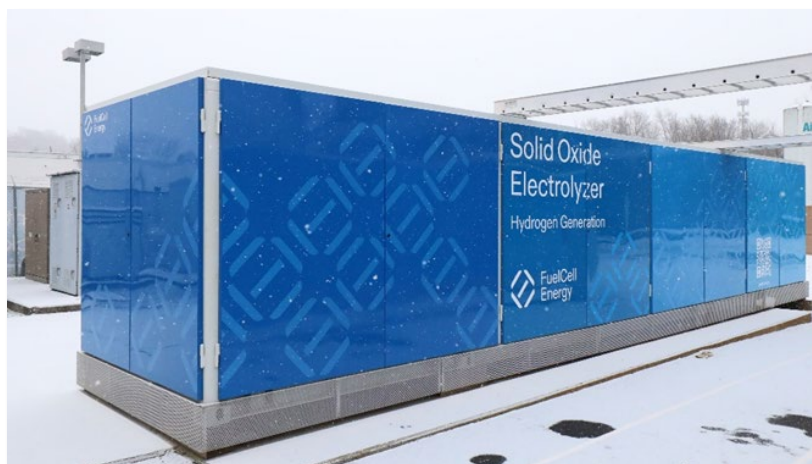
Figure 37 FCE's 150 kg/day SOEC system prototype.
