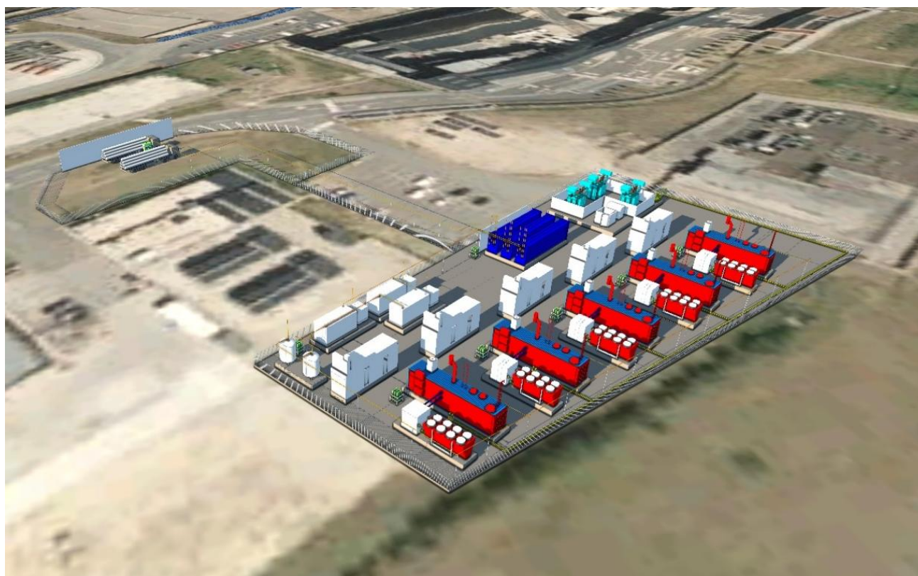
Figure 15: 3D model screenshot of the BBM site, looking north, showing the production area in the centre and dispensing area to the top left
