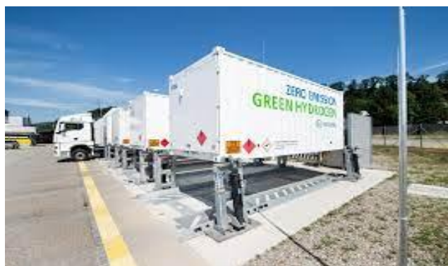
Figure 26: Example MEGC loading bays
