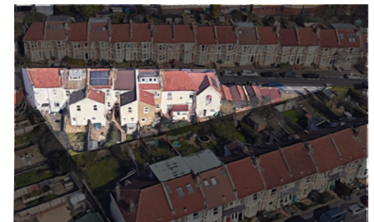
Rear of No's 1-13 + Garages Strathmore Road
