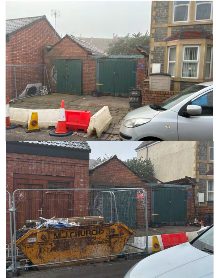
Front of existing Garage
