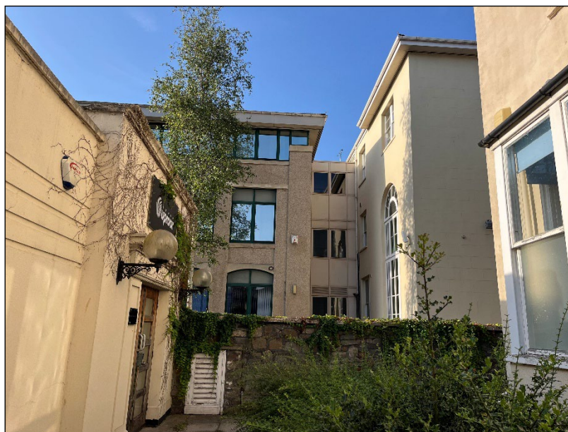
Image 17: Extension to rear of 7 and 9 Whiteladies Road
