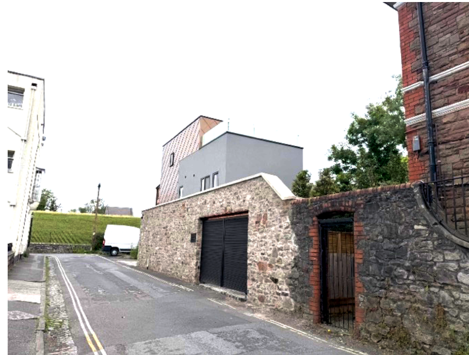
Fig 18: House to the rear of no. 10 St Pauls Road
