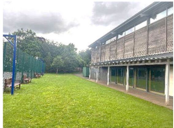
Photograph 6. Southern part of survey area within building B4
