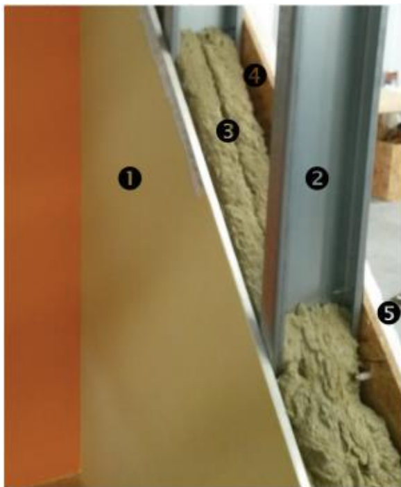
Figure 8. Pictorial view of an LSF wall detail (original figure from [31])
