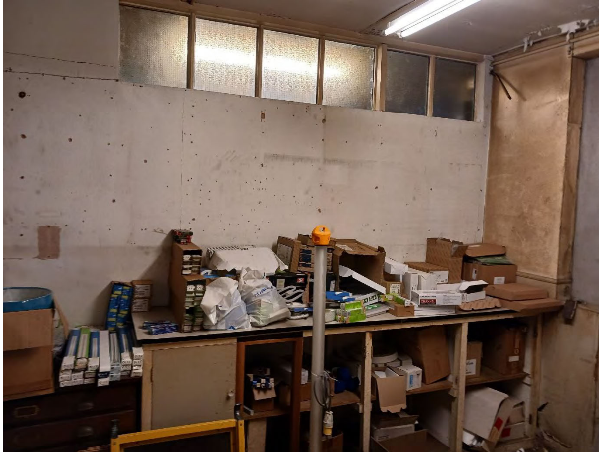
Photo 15 : Dry storage in the existing structure
