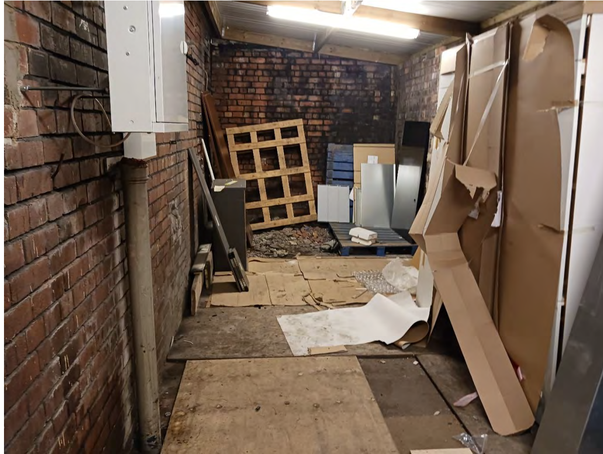
Photo 6: Internal view of existing structure, facing north
