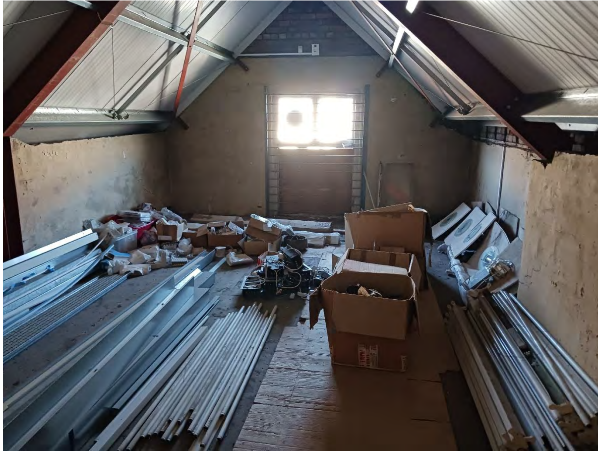
Photo 3 : Internal view of first floor, facing west
