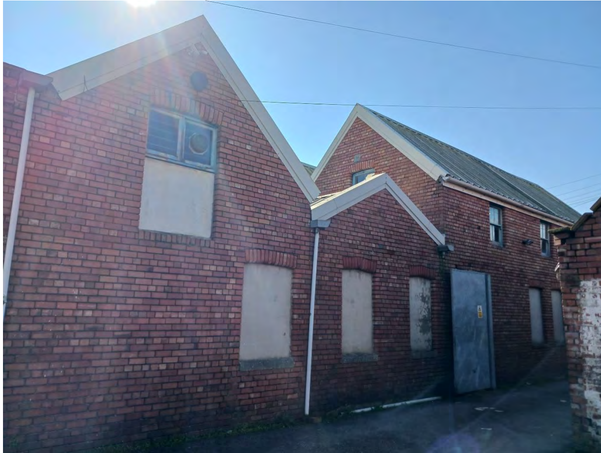
Photo 1: External view of existing structure, facing southeast
