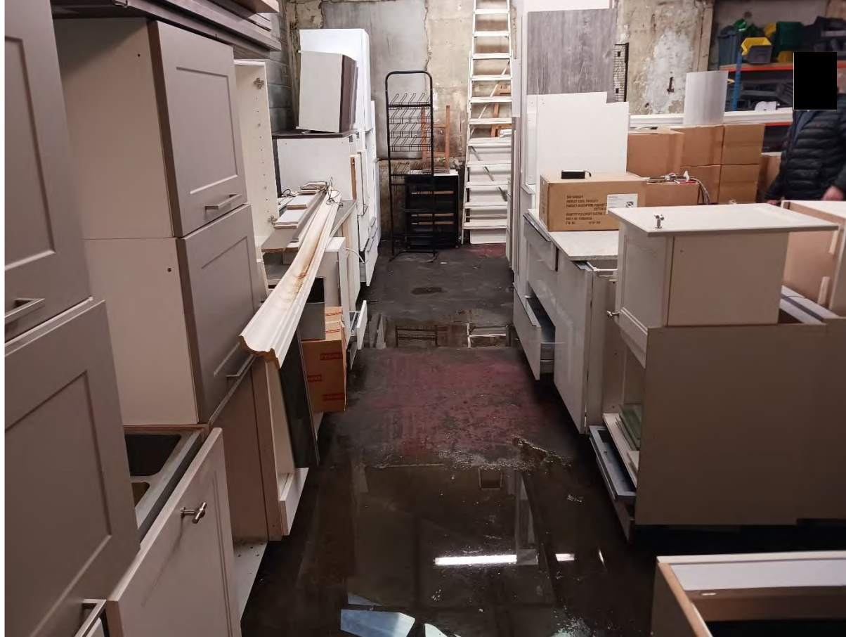
Photo 5 : Internal view of existing structure, facing west
