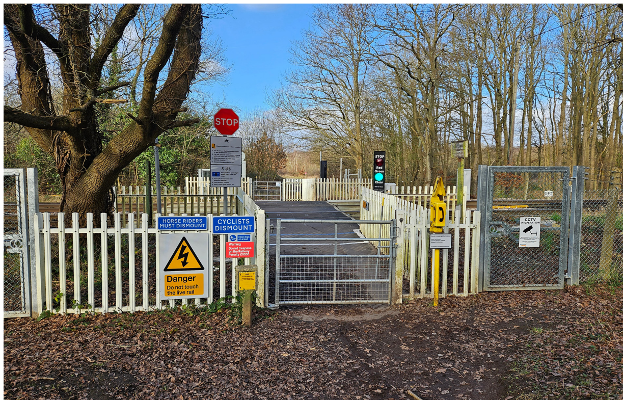
Figure 9: Lady Howard crossing in Surrey, fitted with MSLs and audible warnings.
