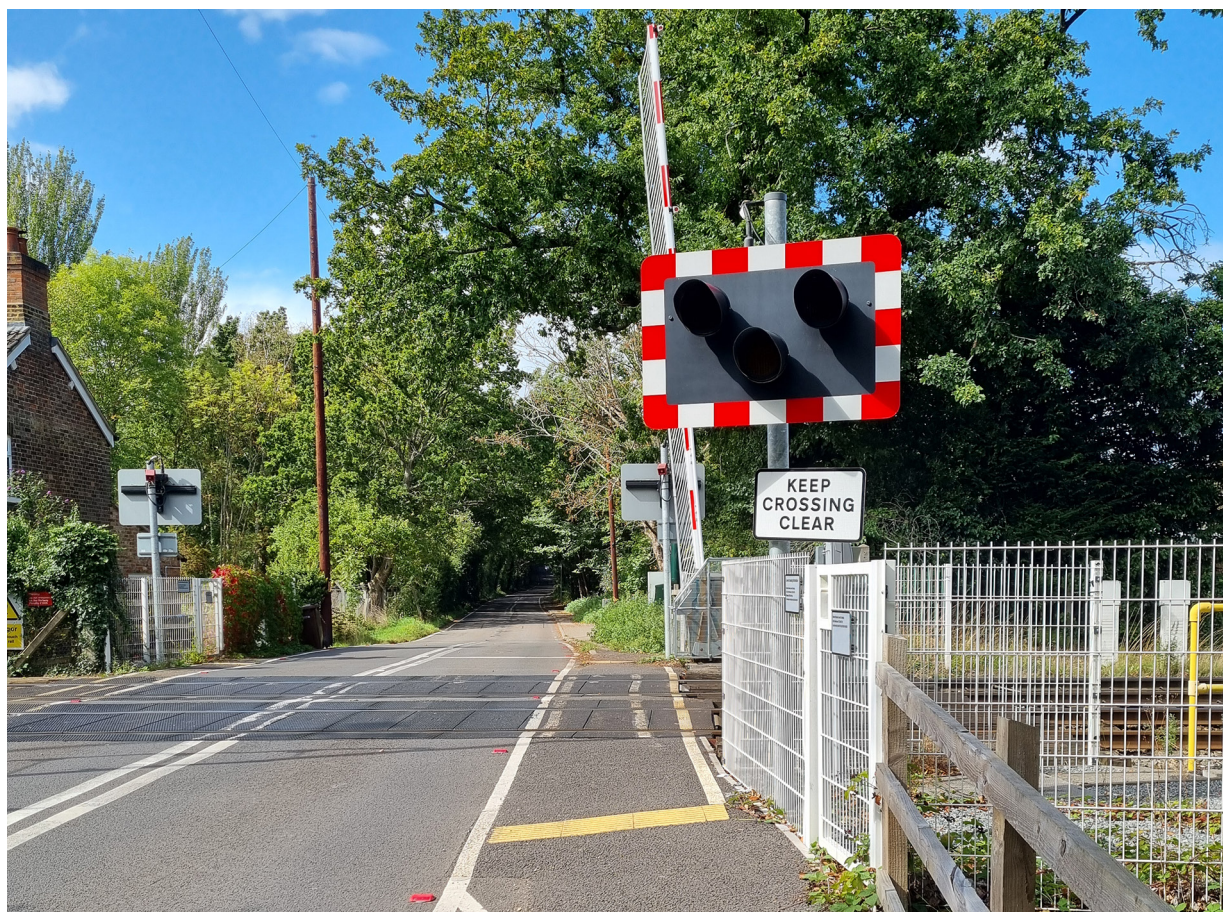
Figure 11: A full barrier crossing, with tactile paving before the barriers.
