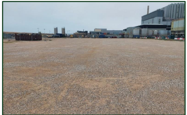
Figure 1 Completed Turbine Hall Basement Infill
