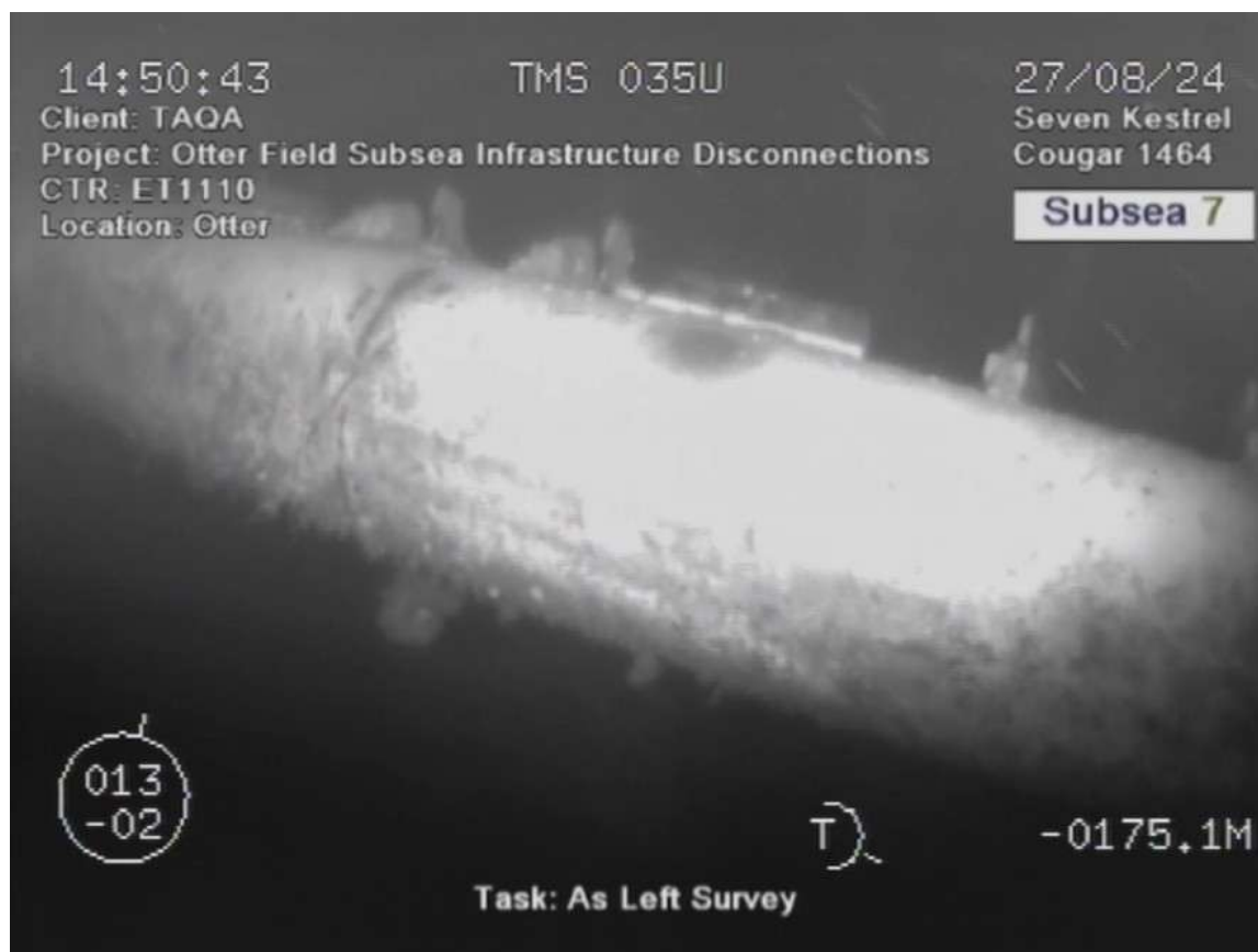
Photograph 2-6: Empty hatches hinges at the Otter template protection structure
