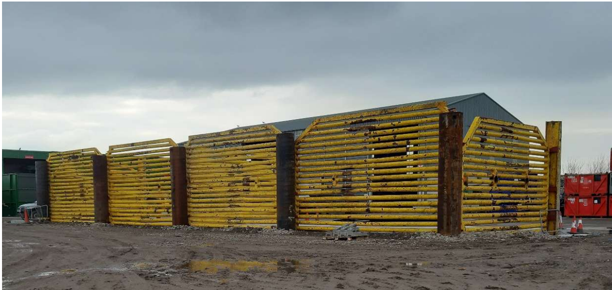
Photograph 5-1: Reuse of seven of the Otter protection structures hatches as a segregation wall at the waste management subcontractor's facilities
