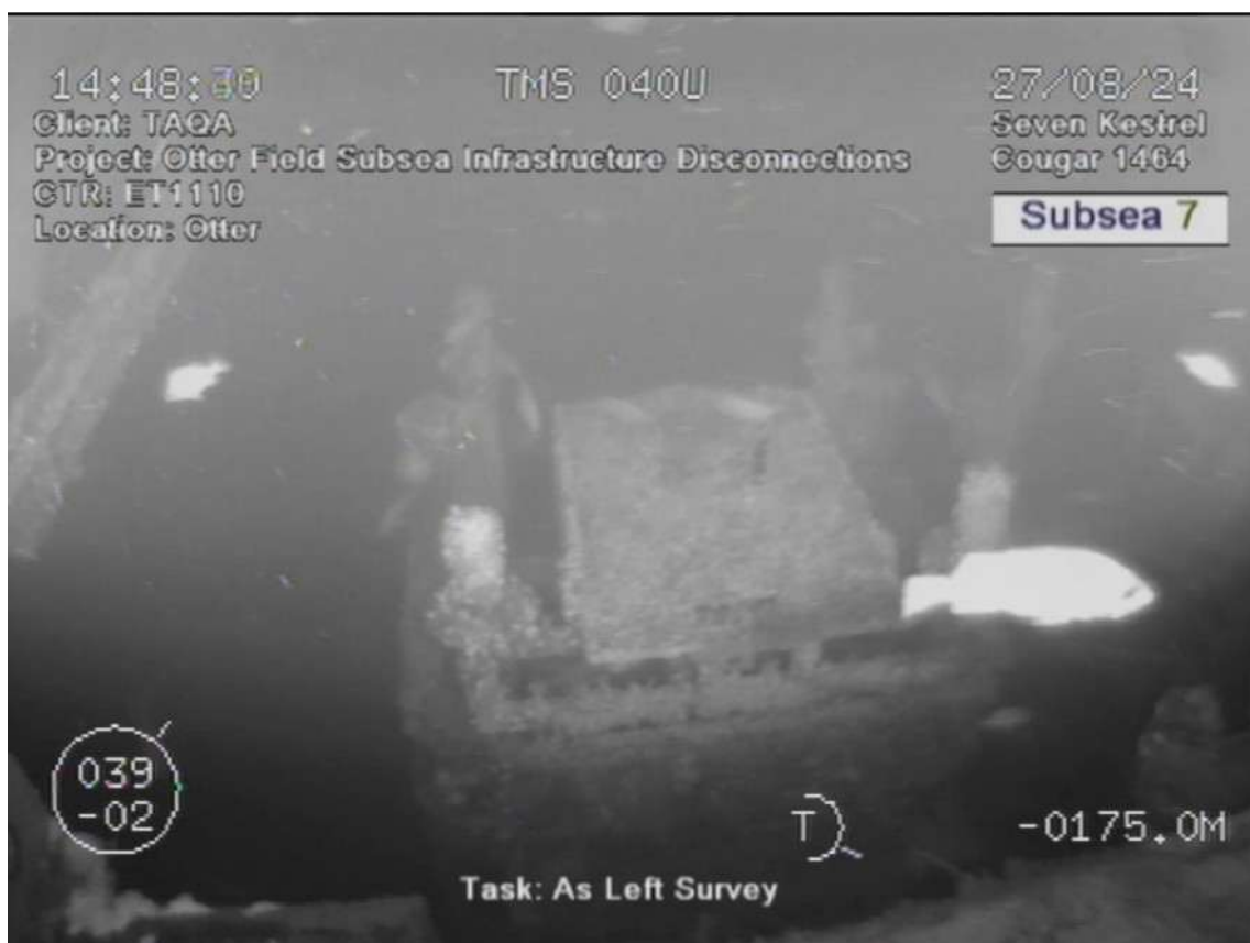
Photograph 2-3: View from the top of the Otter template protection structure showing the Xmas tree below
