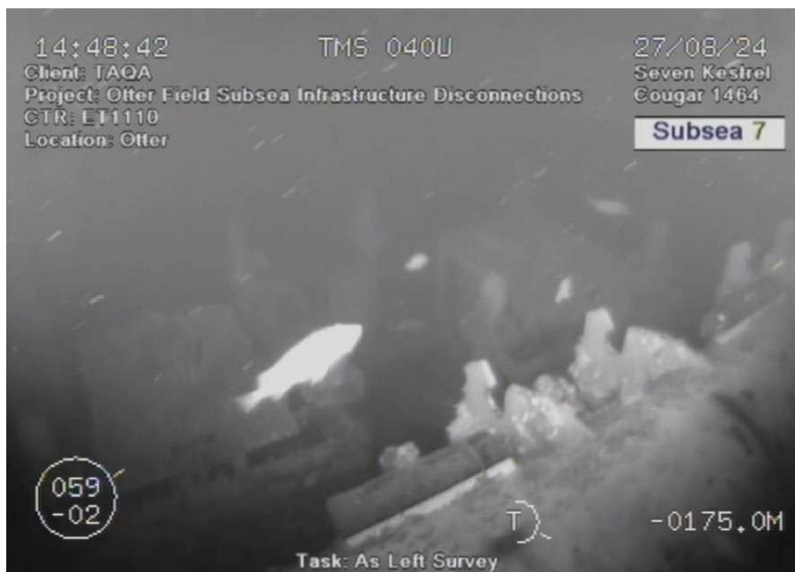
Photograph 2-5: Empty hatches hinges viewed from the top of the Otter template protection structure
