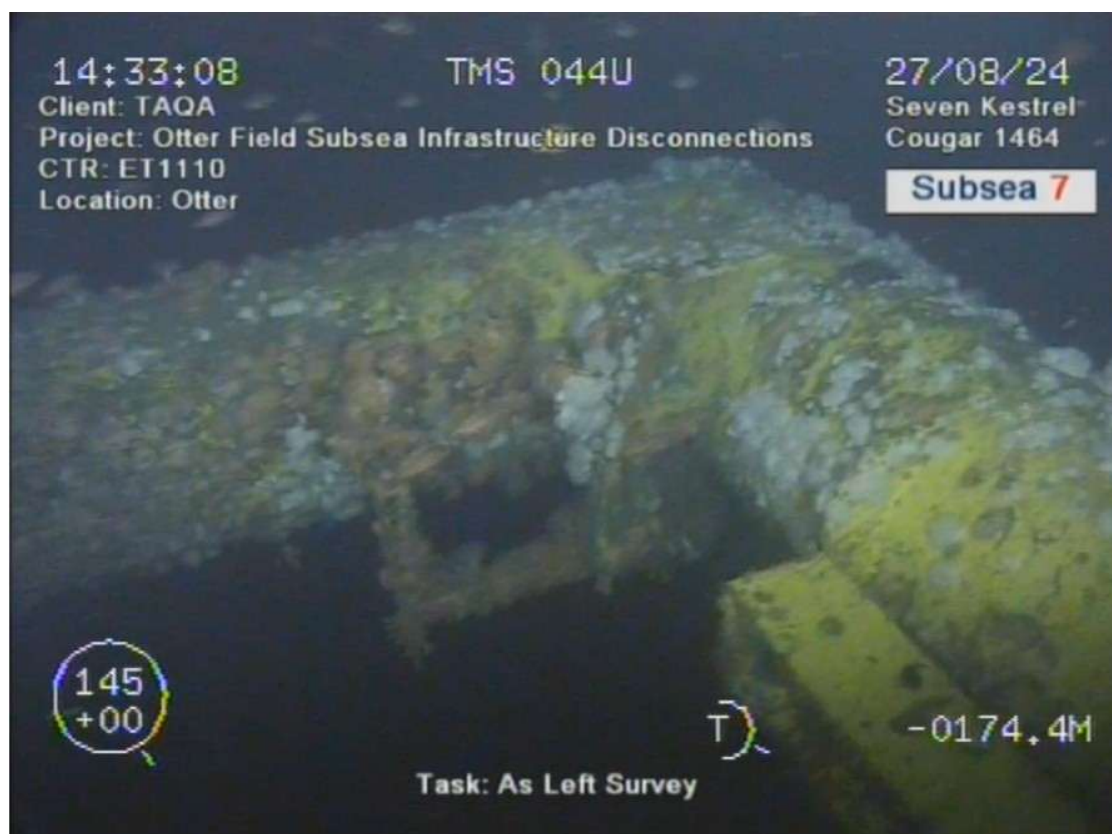
Photograph 2-2: Close up of Otter water injection wellhead protection structure without hatches
