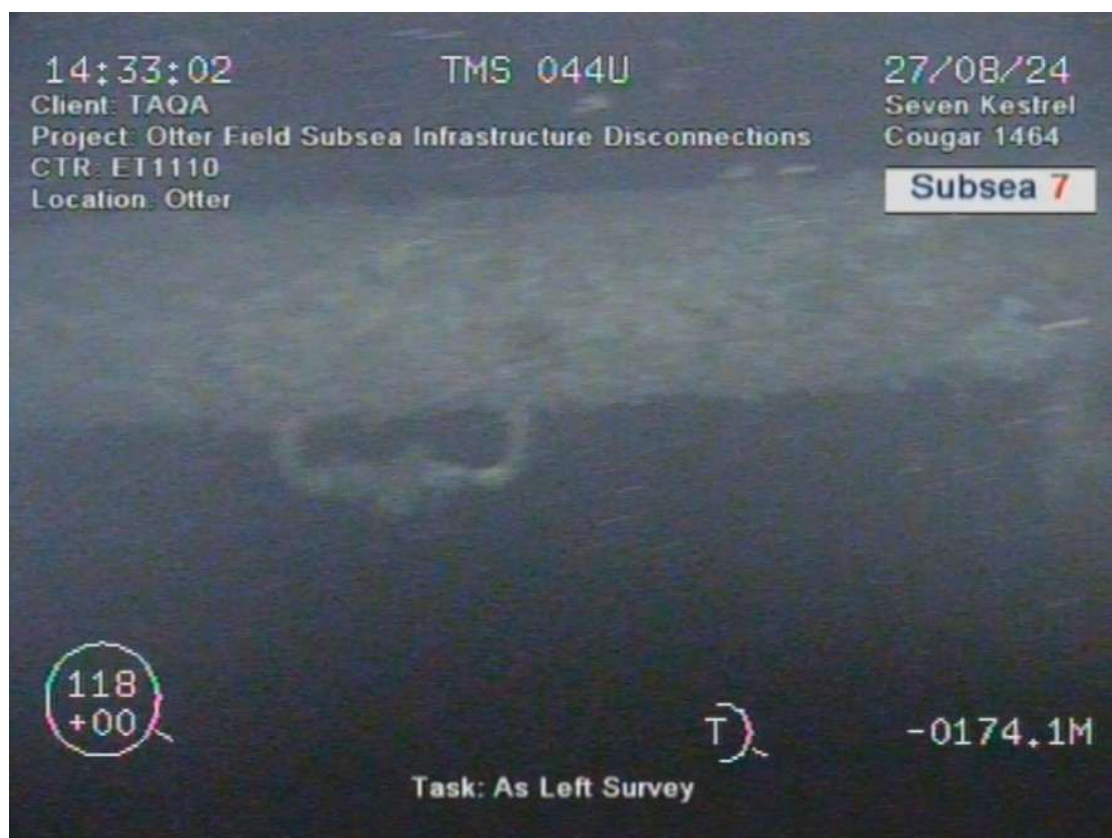
Photograph 2-1: Otter water injection wellhead protection structure without hatches
