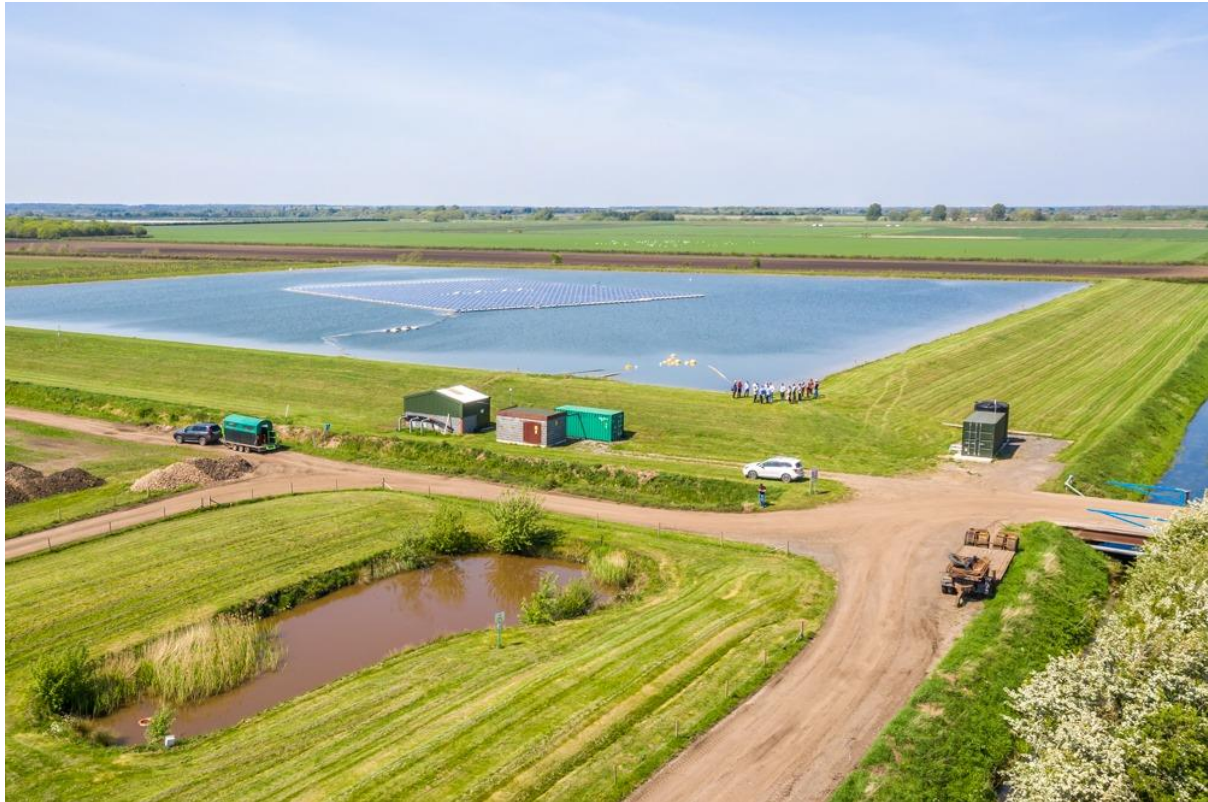
Figure 7.2.6 The Lapwing Estate reservoir with floating solar
