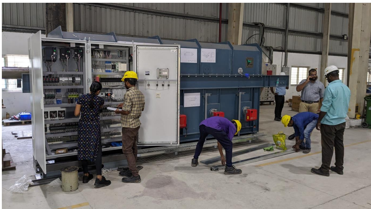
Figure 2.2.2.3. Anergy's team carrying out electrical work on the HTP Kiln electrical panel in Chennai, India
