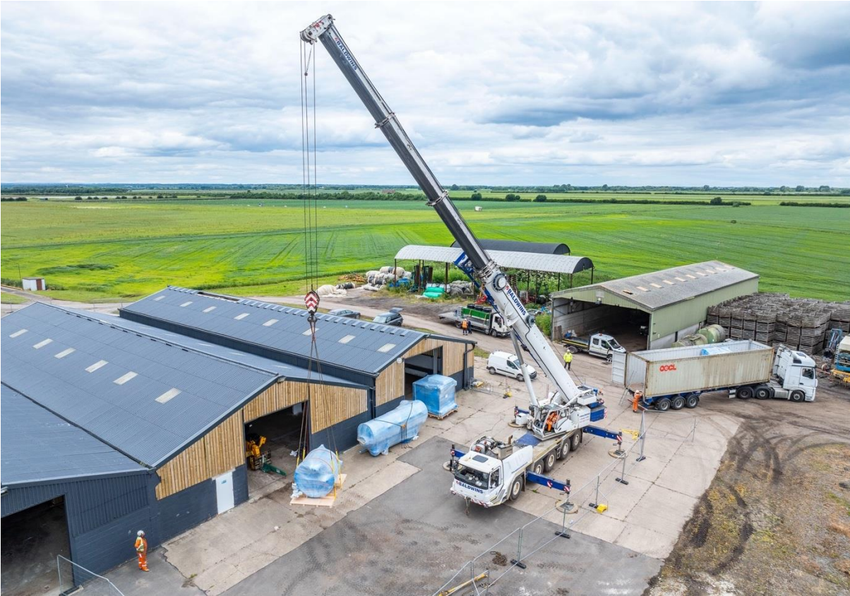
Figure 2.2.3.1. Delivery of the Phase 1 equipment on site
