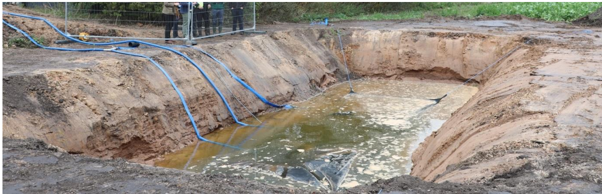
Figure 1.3. Lapwing Energy's patented carbon storage solution
