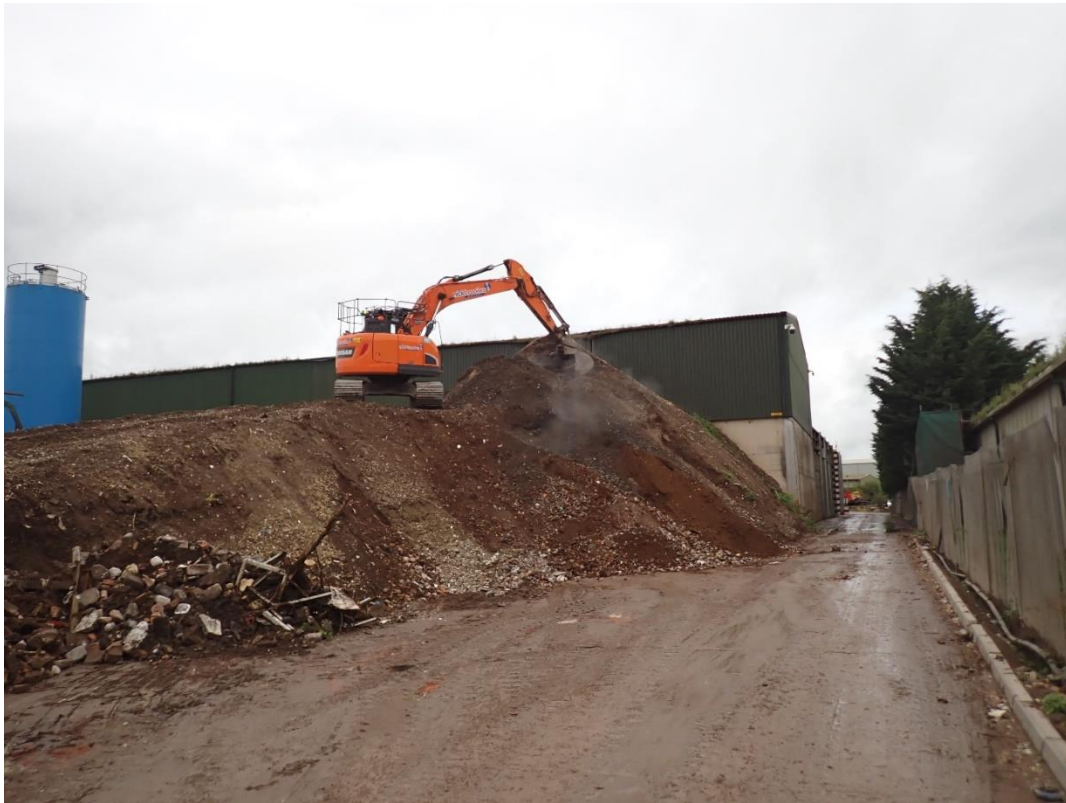
Photograph 3 – Trommel fines steaming on 14/09/2023
