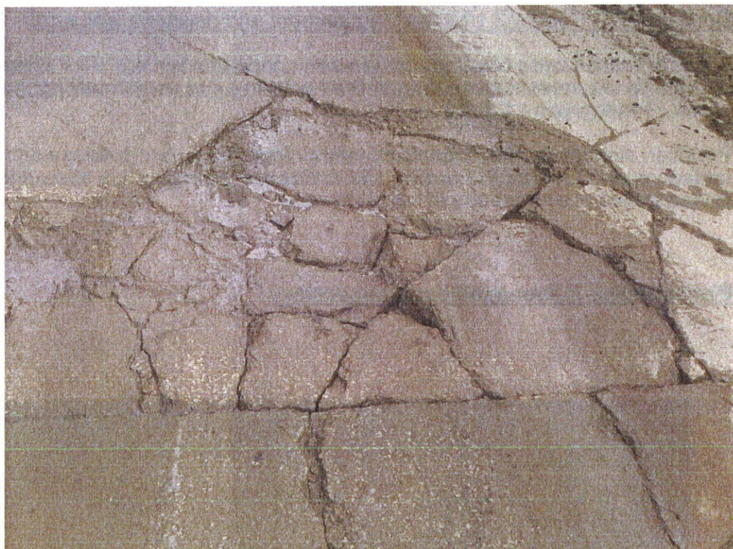
Photograph 3 – Cracked concrete surface. Sprinklers had been operational prior to the inspection as indicated by the wet surface. No mud was noted at the time of the audit to be tracking off site and no dust emissions observed.
