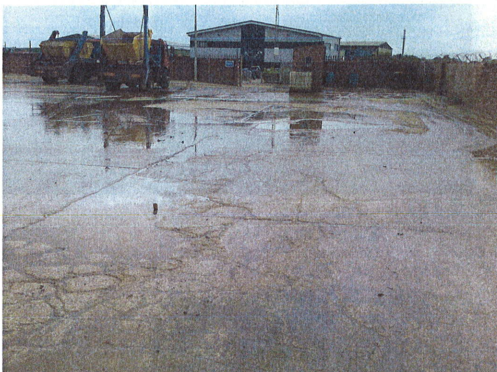
Photograph 3 – Cracked concrete surface. Sprinklers had been operational prior to the inspection as indicated by the wet surface. No mud was noted at the time of the audit to be tracking off site and no dust emissions observed.
