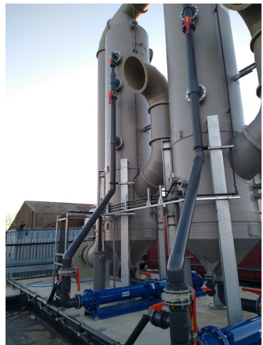
Figure 18: DAC scrubber system
