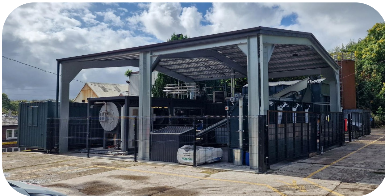
Figure 2 – Ahlstrom Radcliffe site showcasing BBB's PYREG P500 pyrolysis unit, peripheral equipment, canopy and container office.
