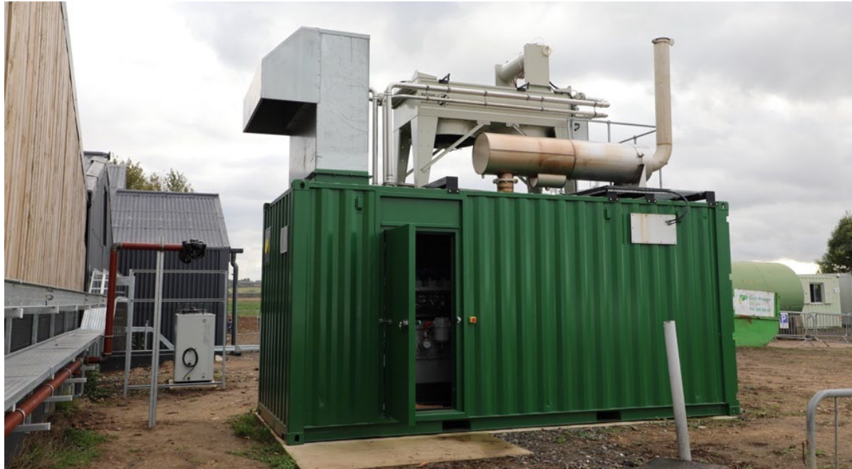
Figure 2.3.1. Gas Engine on site
