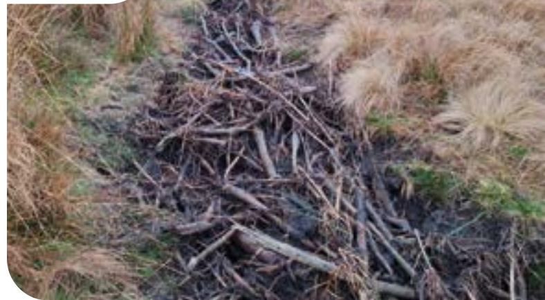
A blocked grip (man-made peatland drainage ditch), to avoid livestock drowning and reduce the wildfire risk of military training © Karen Fisher
