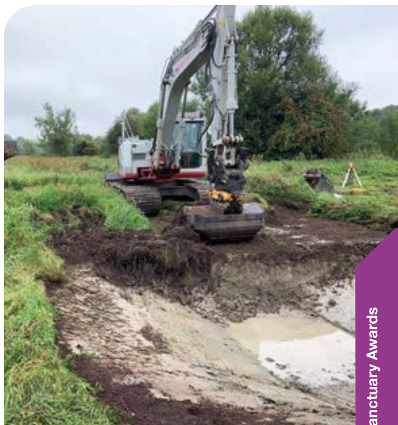
Excavators cutting a new channel © Wiltshire Wildlife Trust
