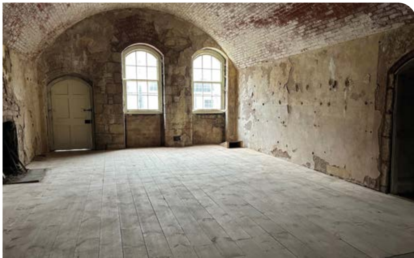
Room with the new suspended timber flooring with bat access in the corner © Crown
