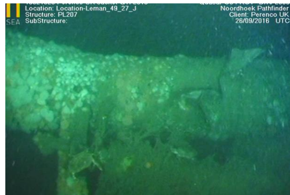
Figure 5: PL207 supported on grout bag [54]
