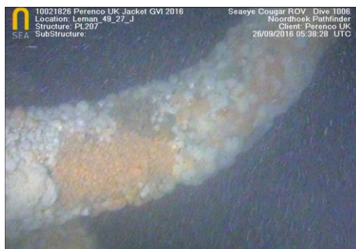
Figure 29: Exposed riser section which continues up to jacket at the back of the structure [54]
