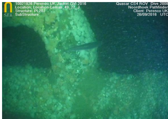
Figure 4: PL207 tee intersection with PL206 [54]
