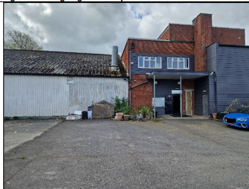
Figure 5. Cement bonded asbestos roofing.
