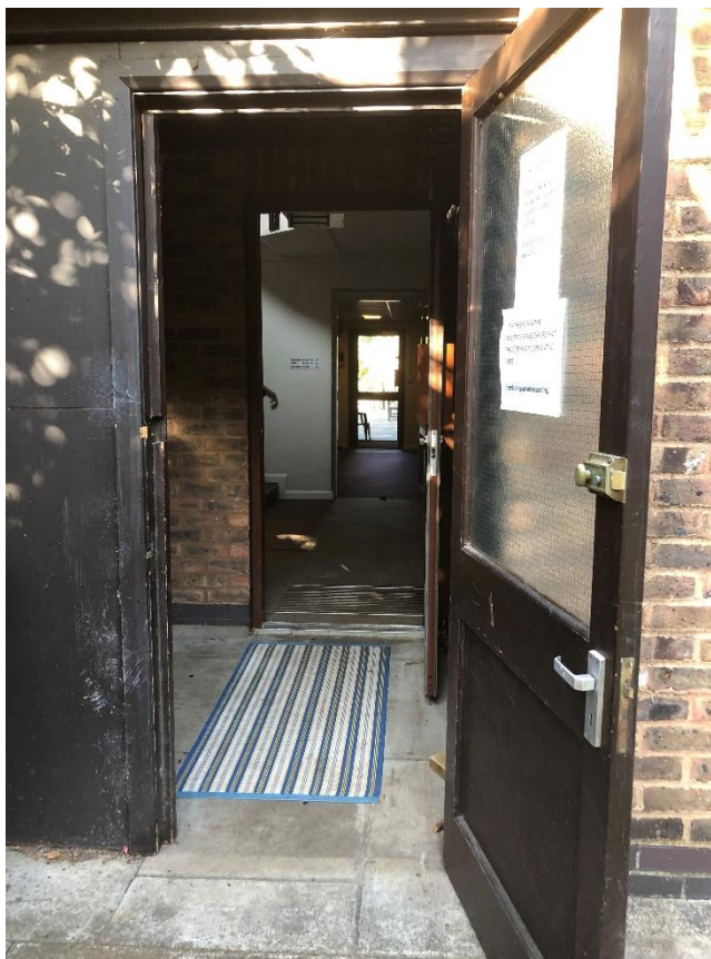
Figure 42 Building 4 images showing under sized store, overspill parking in the escape stair, external door with inappropriate ironmongery
