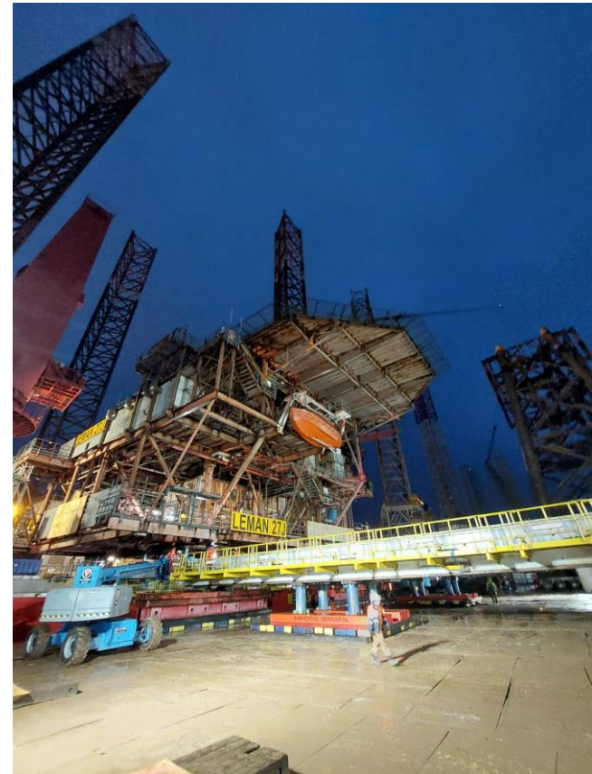
Figure 6: Leman 27J topside being loaded onto the waste disposal yard for dismantlement and waste recovery.
