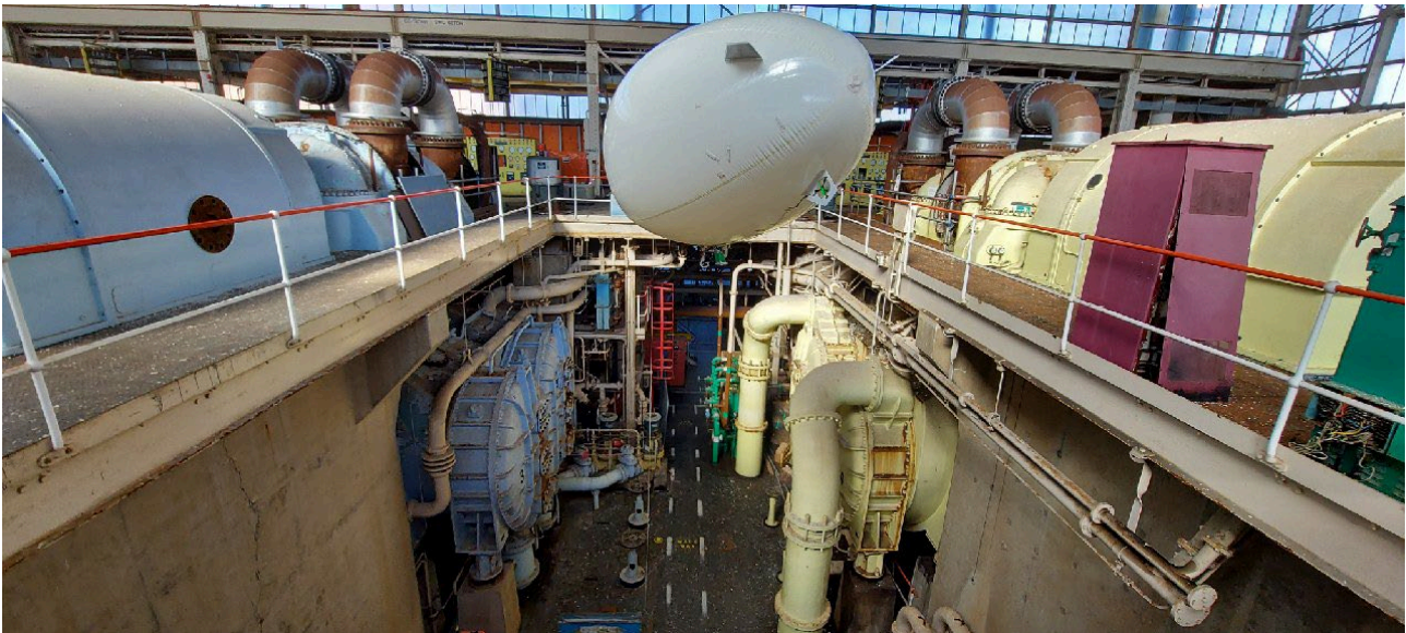
Figure 23: Demonstration of the lighter-than-air inspection vehicle at a facility on the Sellafield nuclear site (image supplied by Sellafield Ltd).
