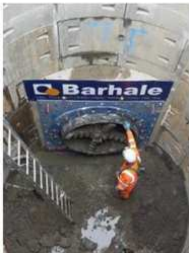
Figure 3 Representative 4m reception shaft being entered by an MTBM
