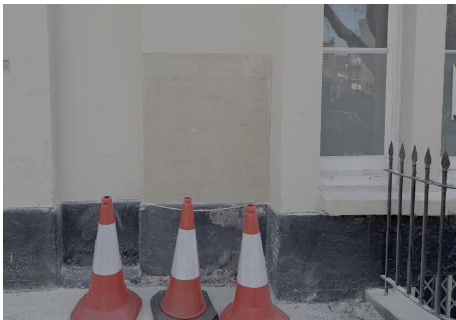
Fig 10: Test patch for the removal of the paint finish showing the Bath Stone surface behind
