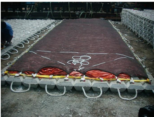
Figure 2.4.18: Typical concrete and concrete fronded mattresses (6m x 3m x 0.15m)
