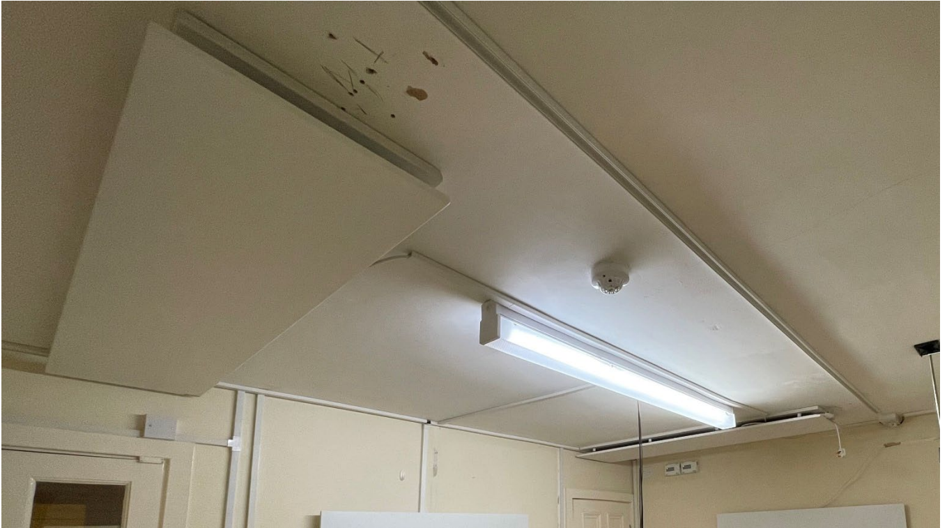
Figure 2-6 IR Heater type 2 installed in Room A
