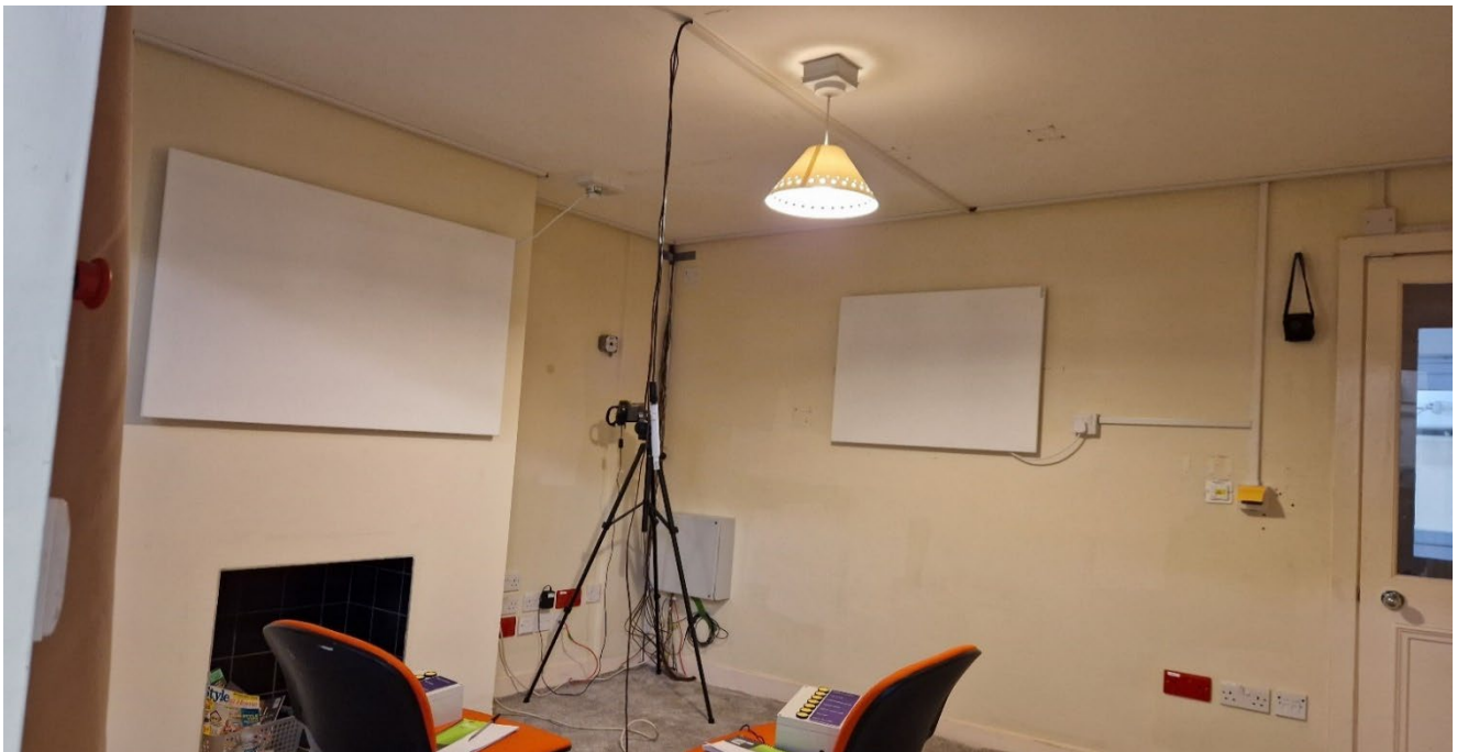
Figure 2-5 IR Heater type 1 installed in Room B
