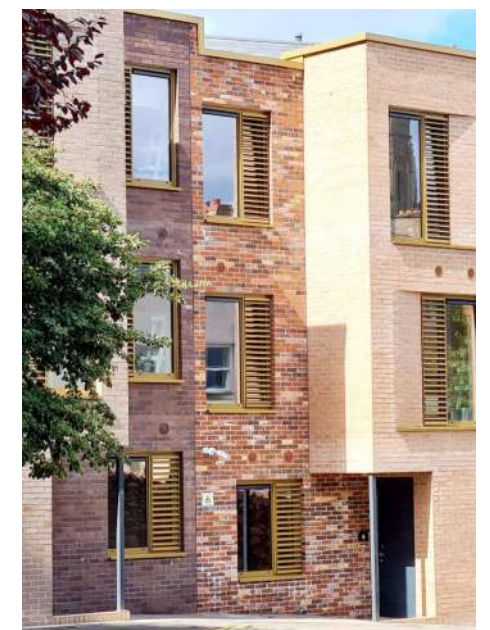
Fig. 38 Example of louvred windows - St Mary's Student Accommodation, Bristol (Architectural Aluminium and Glass Ltd.),
