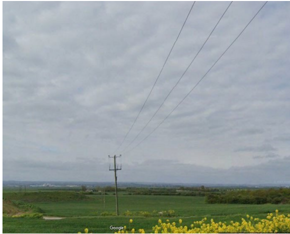
Figure 6: Examples of 6.6 kV three-phase overhead lines
