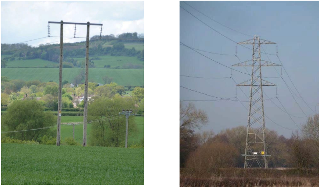
Figure 13 (Left) Photo of a 66 kV wooden pole overhead line (Right) Photo of a 132 kV steel lattice pylon
