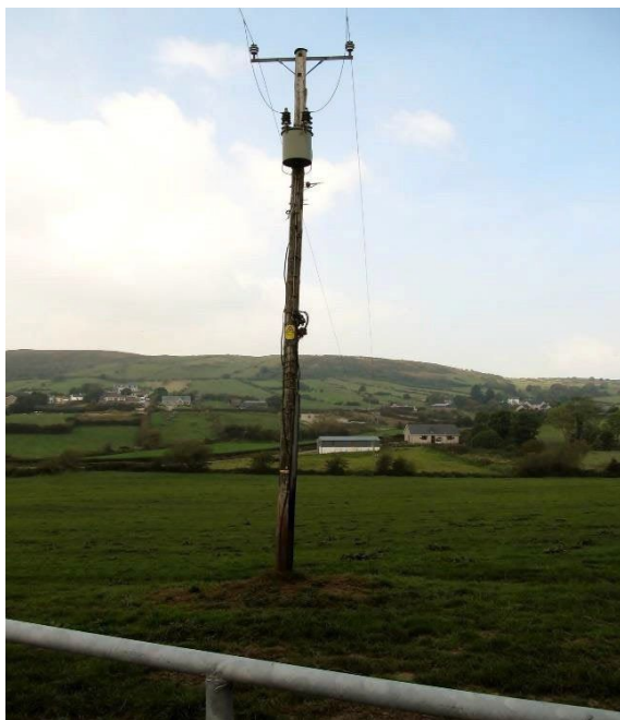
Figure 5: (Left) A single phase circuit (Right) A three-phase single circuit line
