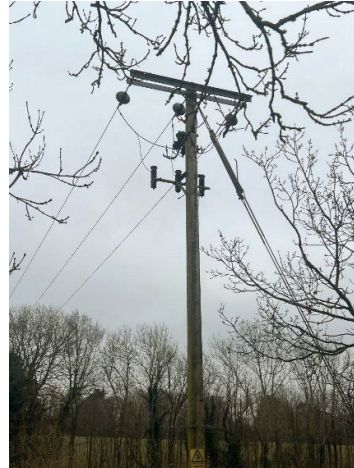
Figure 6: Examples of 6.6 kV three-phase overhead lines
