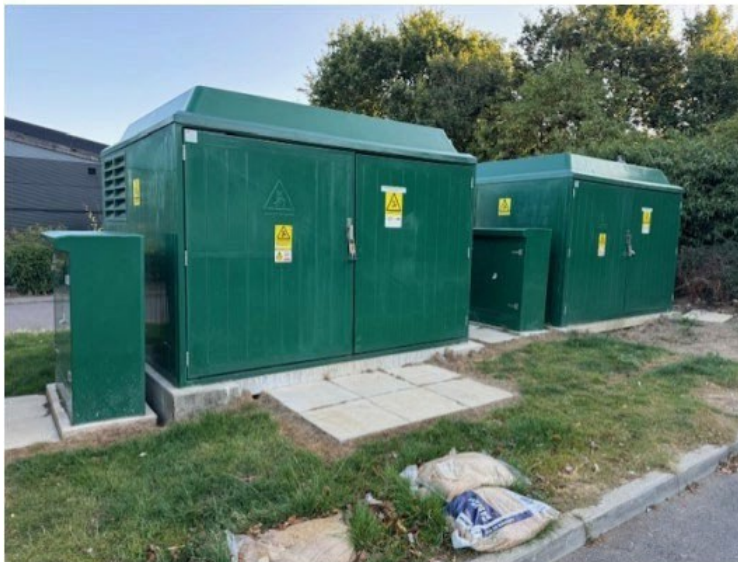
Figure 2: Two substations installed next two each other to provide capacity for electric vehicle charge point supply at a motorway service station. 17
