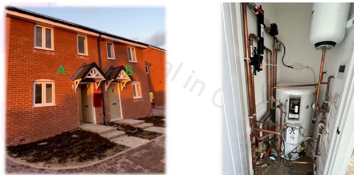
Figure 3: Trial site installation. The heat pump system on the right is housed in building A, building B contains a conventional heat pump system.
